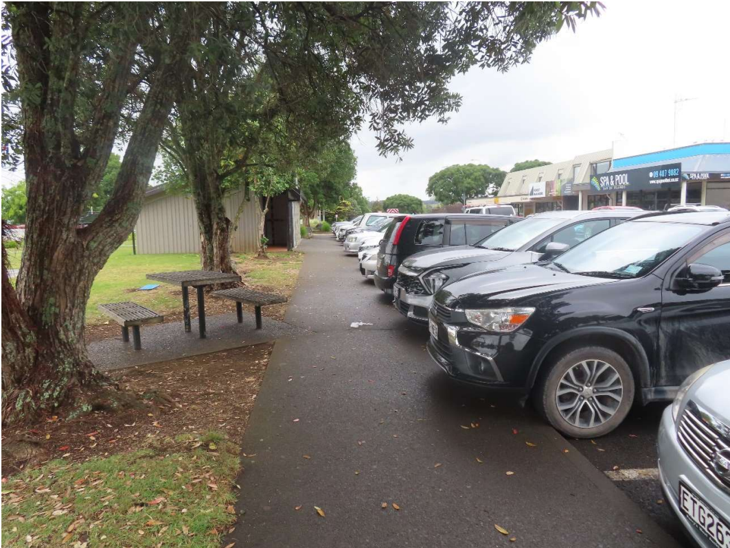
Figure 2 ; Kerikeri Domain, narrow footpath with overhanging vehicles limiting effective width of footpath. Two mobility scooters would struggle to pass.
