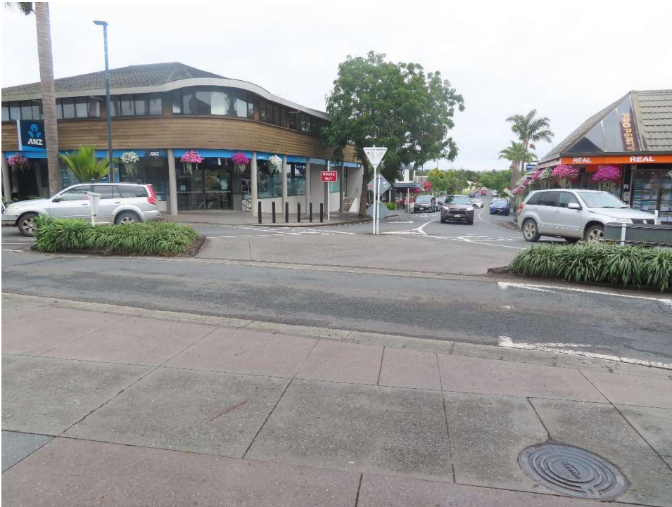
Figure 6 : Intersection of Fairway Drive and Kerikeri Road showing absence of formal crossing facilities.
