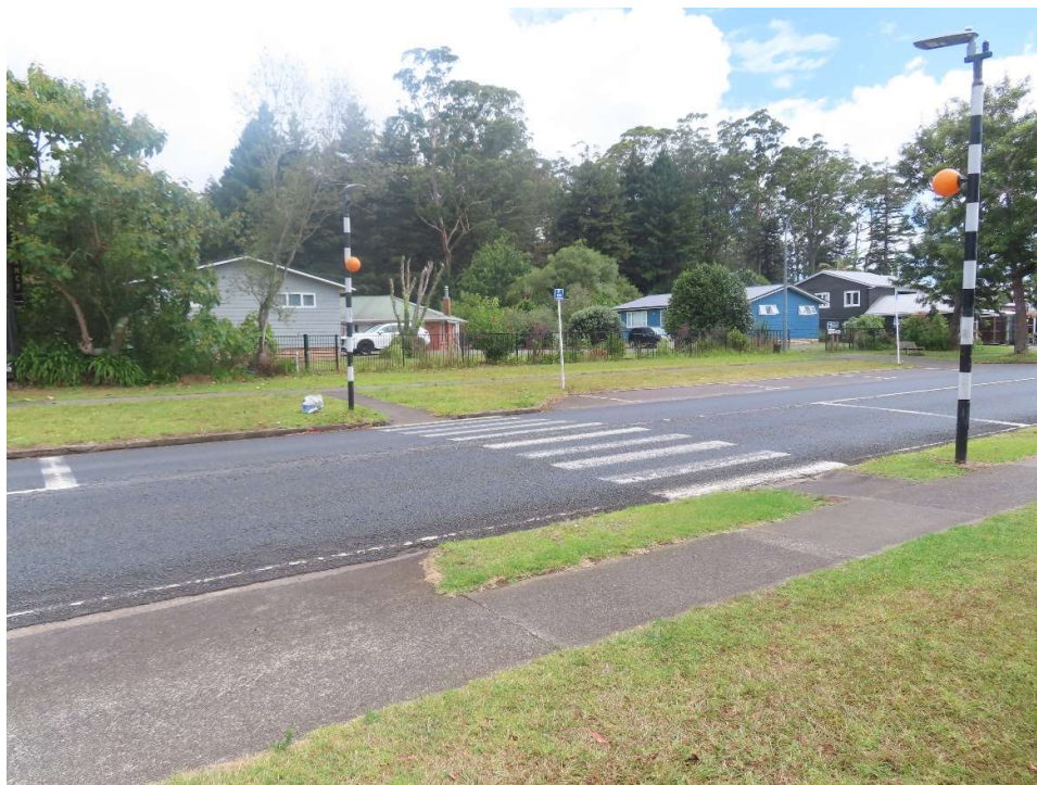
Figure 7 : Crossing of Kerikeri Road showing poor facilities and ride for wheeled devices.
