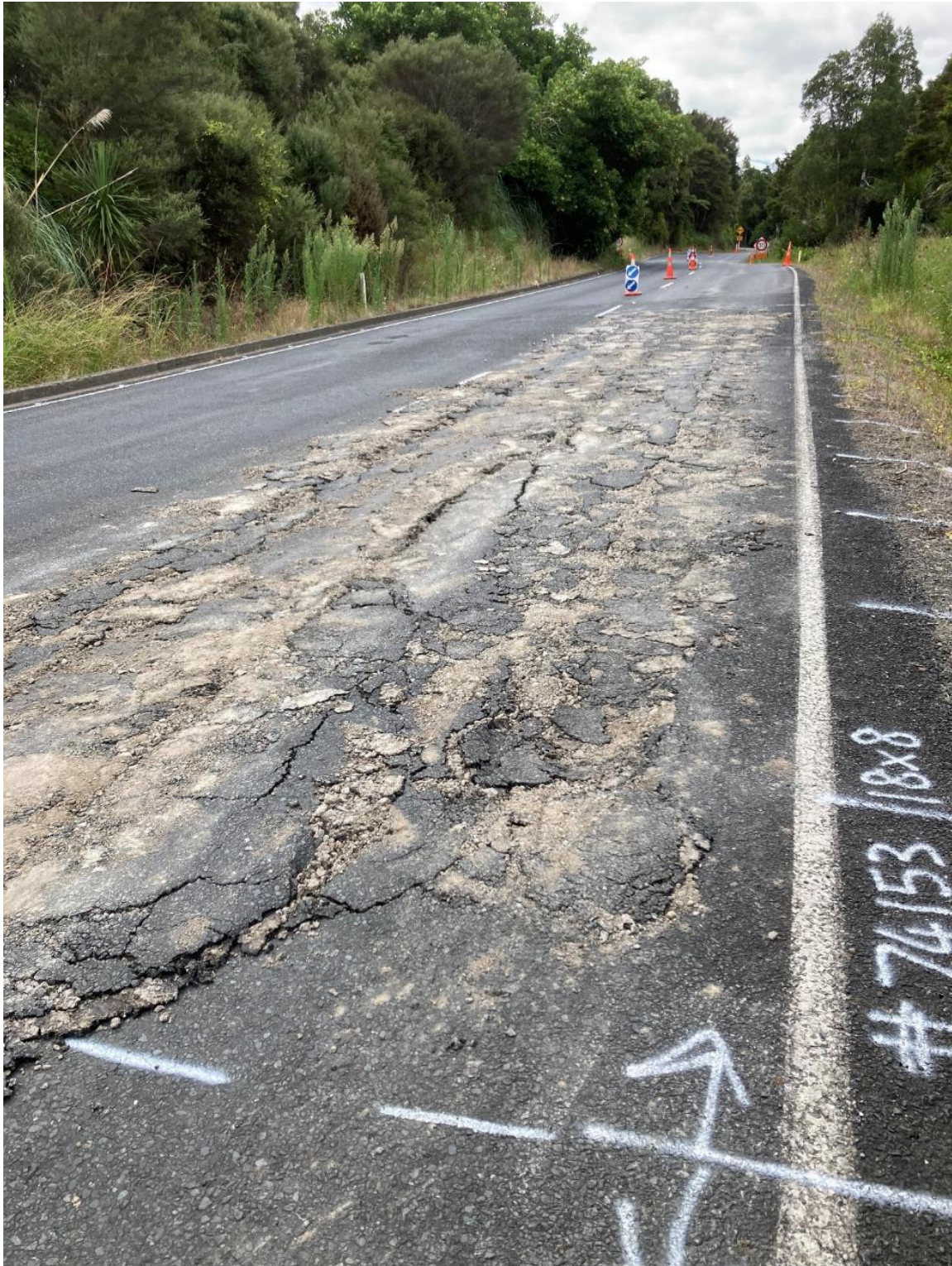
Pre reseal repair ready for stabilising on West Coast Rd
