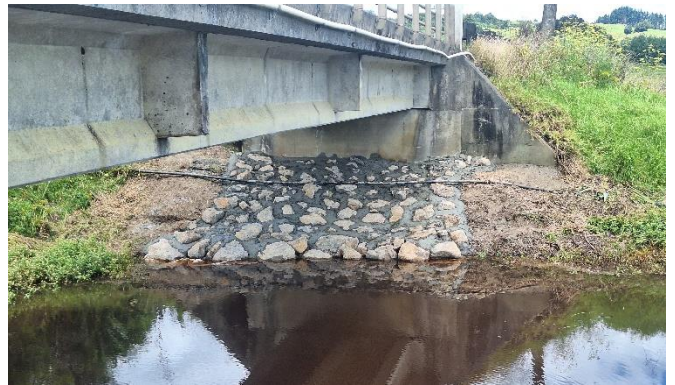
7/21/215 SP3 – Scour Protection Works at Pokapu Road Bridge T05 (South Abutment)
