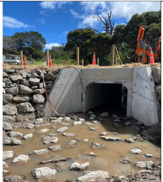
7-23-102 Whangaroa, Waharua & West Coast Road Culvert Renewals (Waharua Rd)
