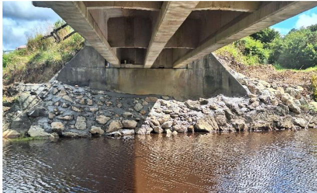
7/21/215 SP3 – Scour Protection Works at Pokapu Road Bridge T05 (North Abutment)
