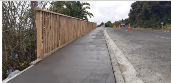
Cable Bay Block Rd 2 nd retaining wall with handrail and fresh pour before washing for exposed aggregate.
