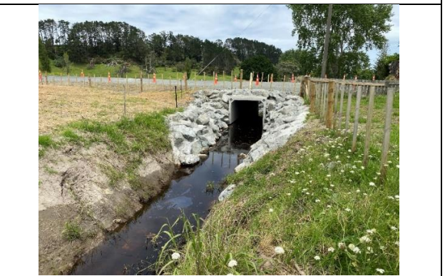
7/23/101 Quarry Road B13 Culvert Replacement
