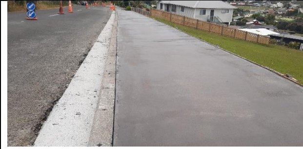
Cable Bay Block Rd fresh pour before washing for exposed aggregate
