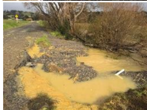
Before/After Tipene Rd Culvert Renewal
