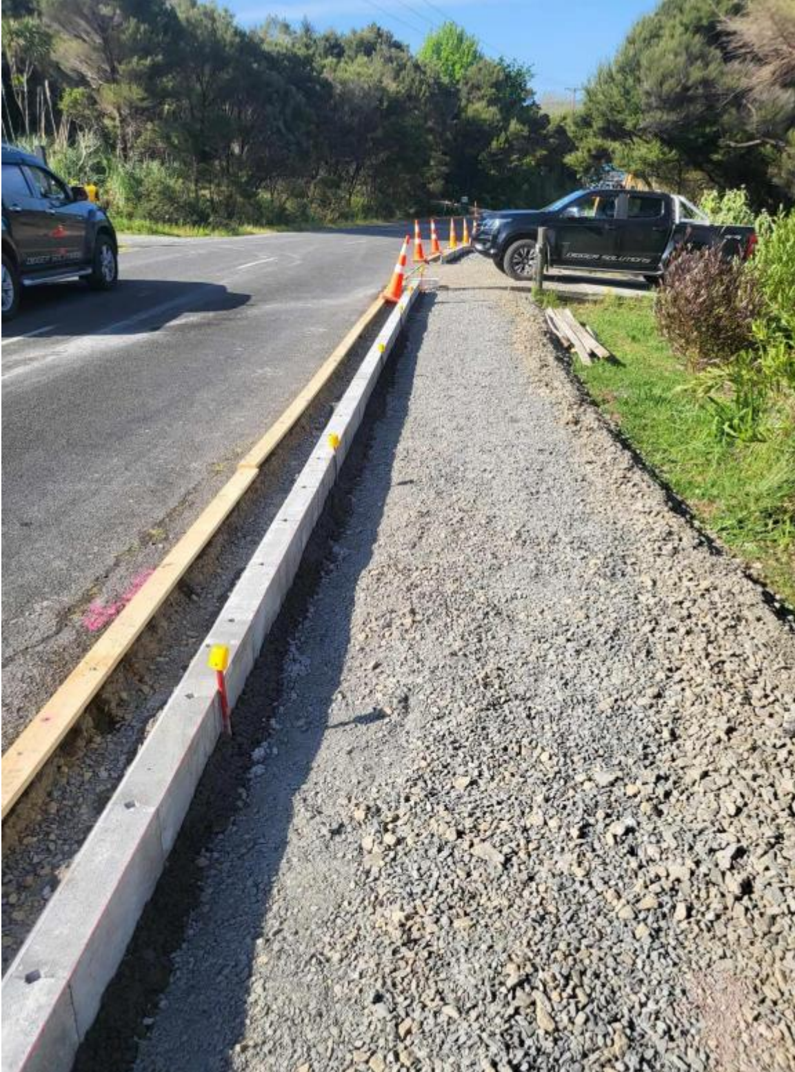
Cable Bay Block Road New Footpath Prep
