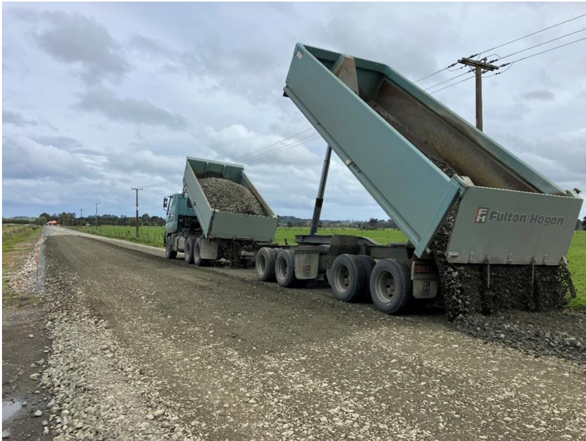
Gill Rd Pavement Rehabilitation Overlay
