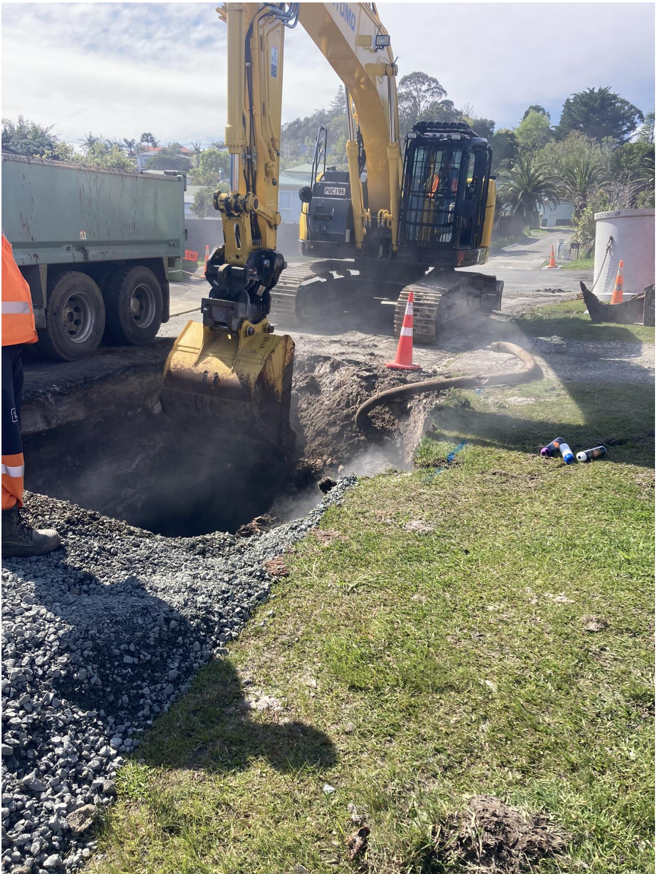
Sommerville Ave SW Upgrade Installation
