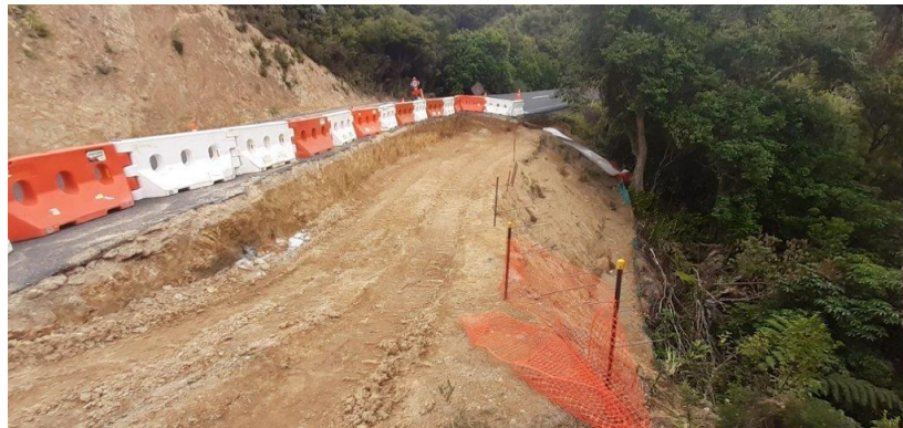
Contract 7/22/150 - FNDC Slip Repairs Suite 01
