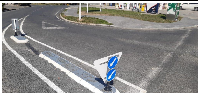
Contract 7/21/216 - Corridor & Intersection Safety Treatments
