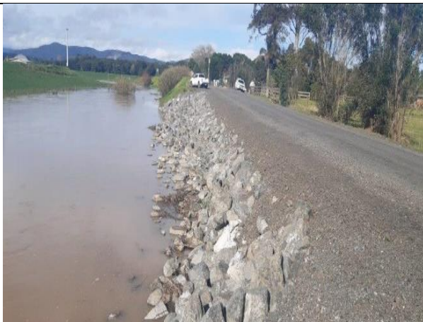
Gill Road – Completed profiled rock wall retaining structure
