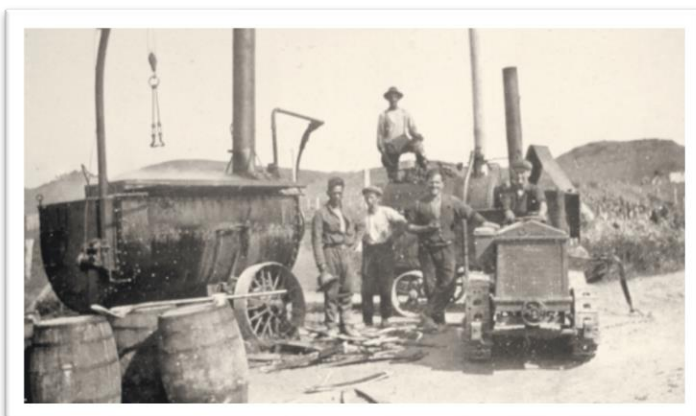
Horse drawn bitumen sprayer ready for sealing the main street of Opunake (right side photo)
