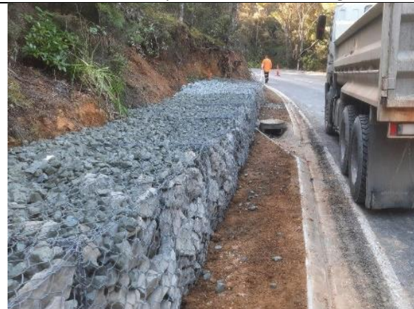
Gabion Wall (Cove Rd RP16,000)
