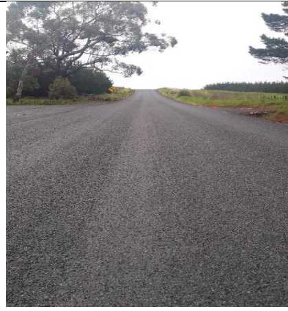
2 nd coat reseals on Pouto seal extension
