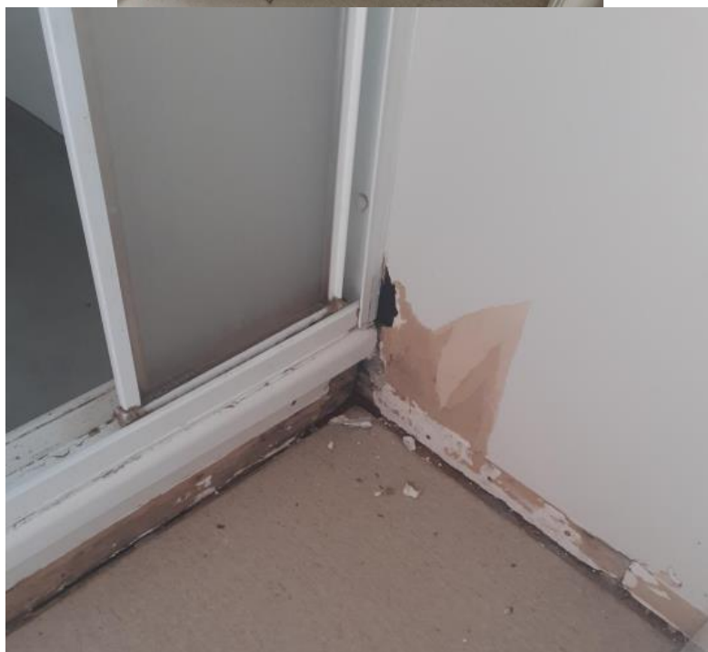
Unit 2, Waima washtub removed, damaged wall lining, and flooring replaced
