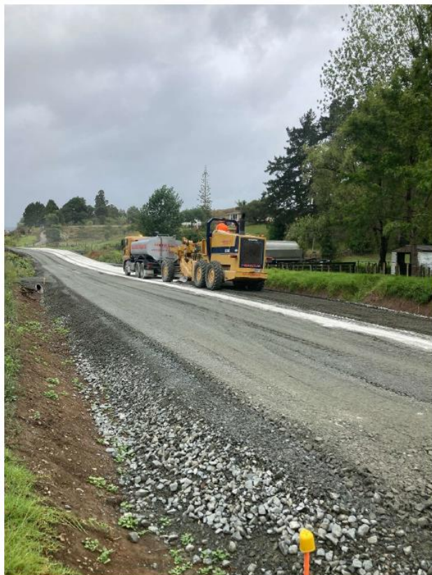
Figure 6: Oruru Rd Rehabilitation Site 2 Stabilising
