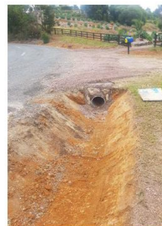
Valencia Lane – 18m of culvert replacement
