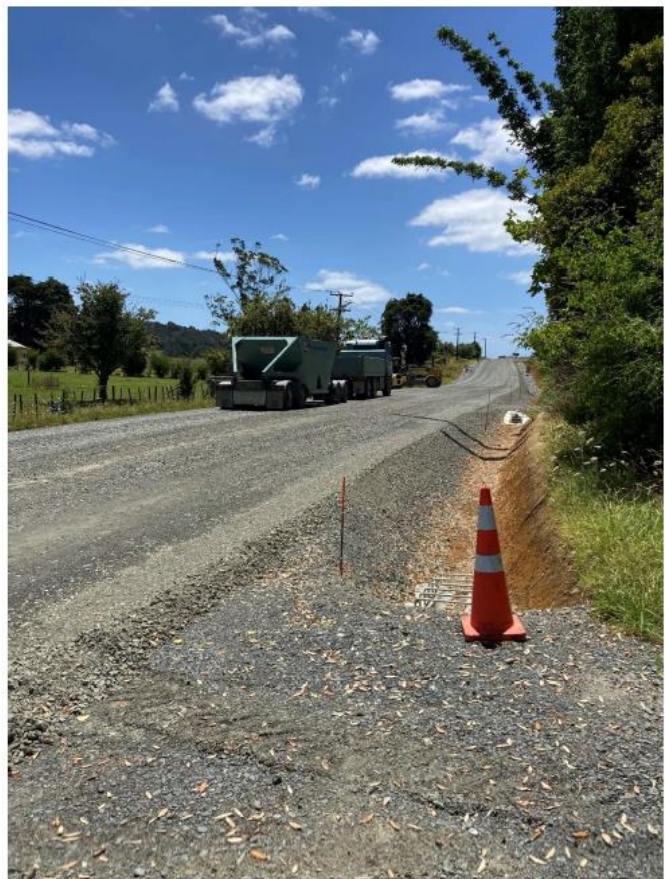
Figure 10: Oruru Rd Rehabilitation Site 1 Pavement Overlay
