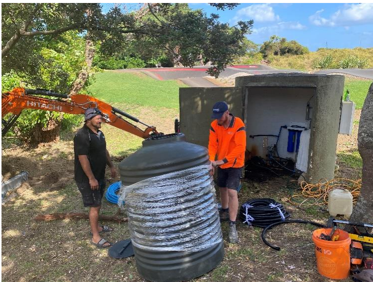
New tank being installed to increase pressure
