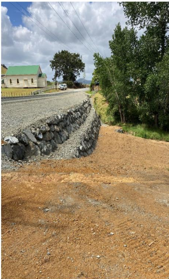
Figure 9: Oruru Rd Rehabilitation Site 1 Rockwall Widening Complete
