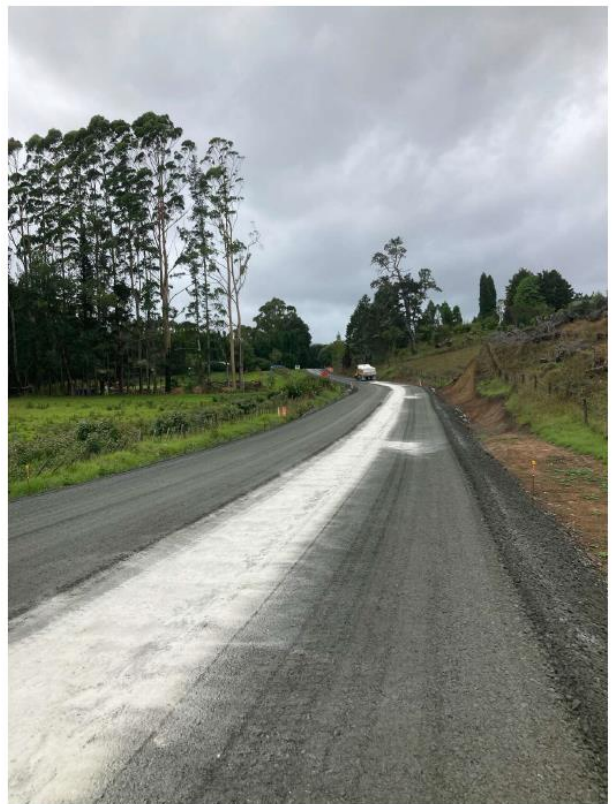
Figure 5: Oruru Rd Rehabilitation Site 2 Stabilising
