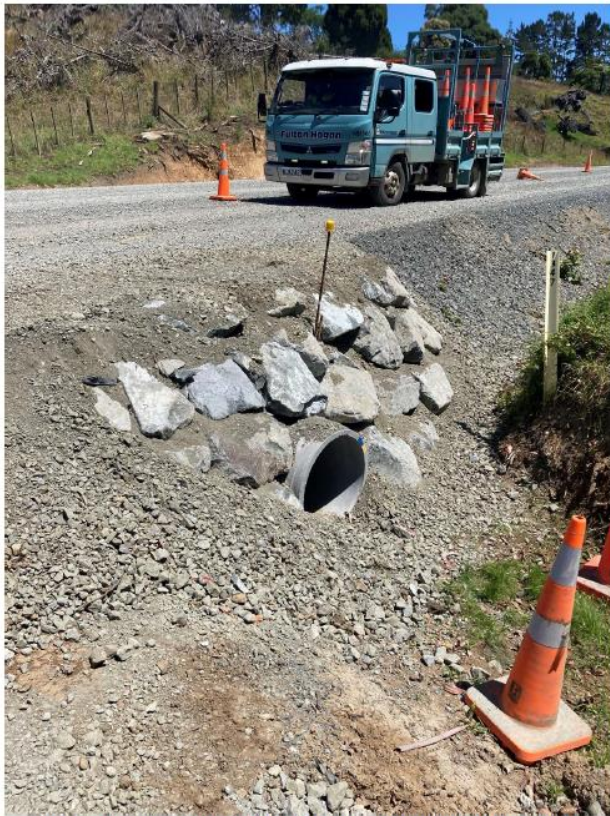
Figure 4: Oruru Rd Rehabilitation Site 2 Headwall Construction
