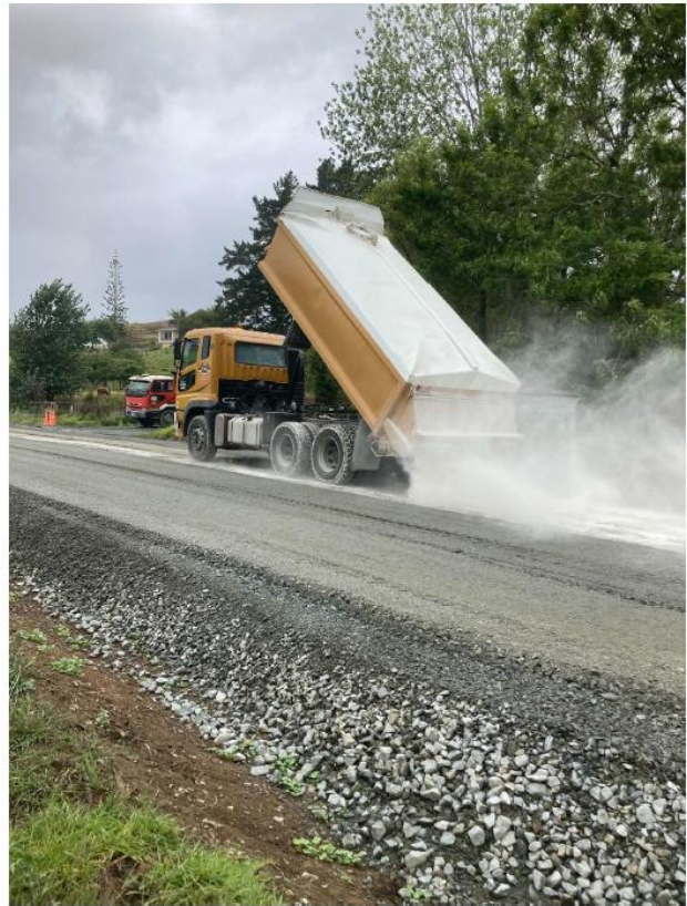
Figure 5: Oruru Rd Rehabilitation Site 2 Stabilising
