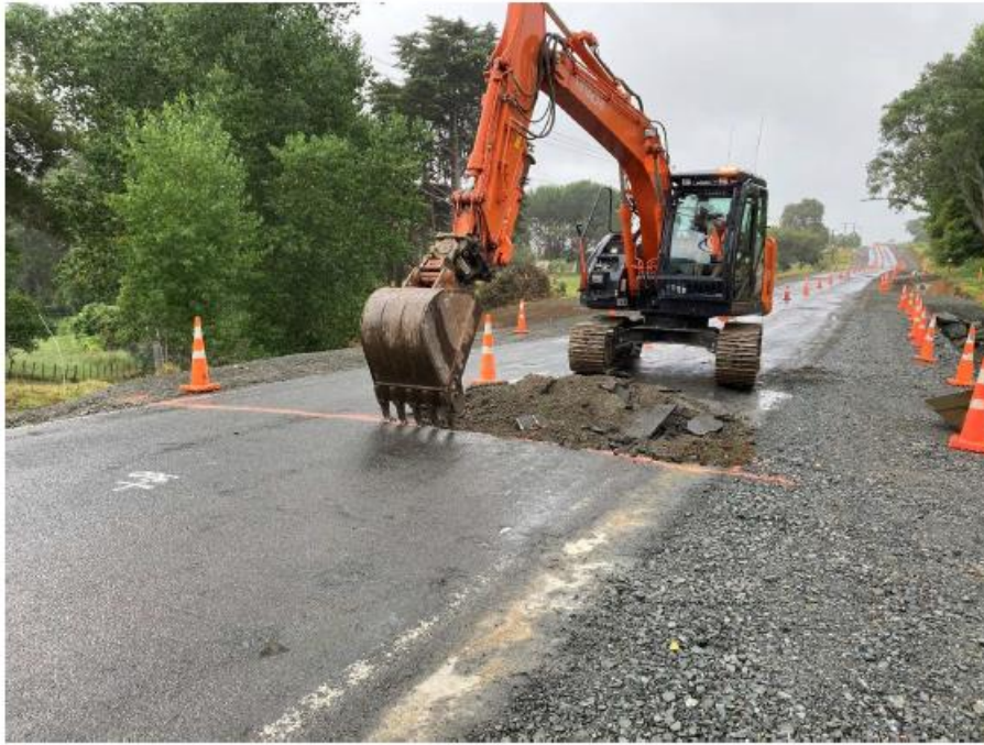
Figure 8: Oruru Rd Rehabilitation Site 1 Pavement Tie-ins
