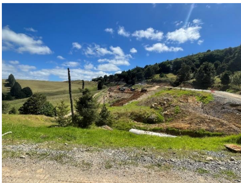
2100 diameter culvert pipe installed
