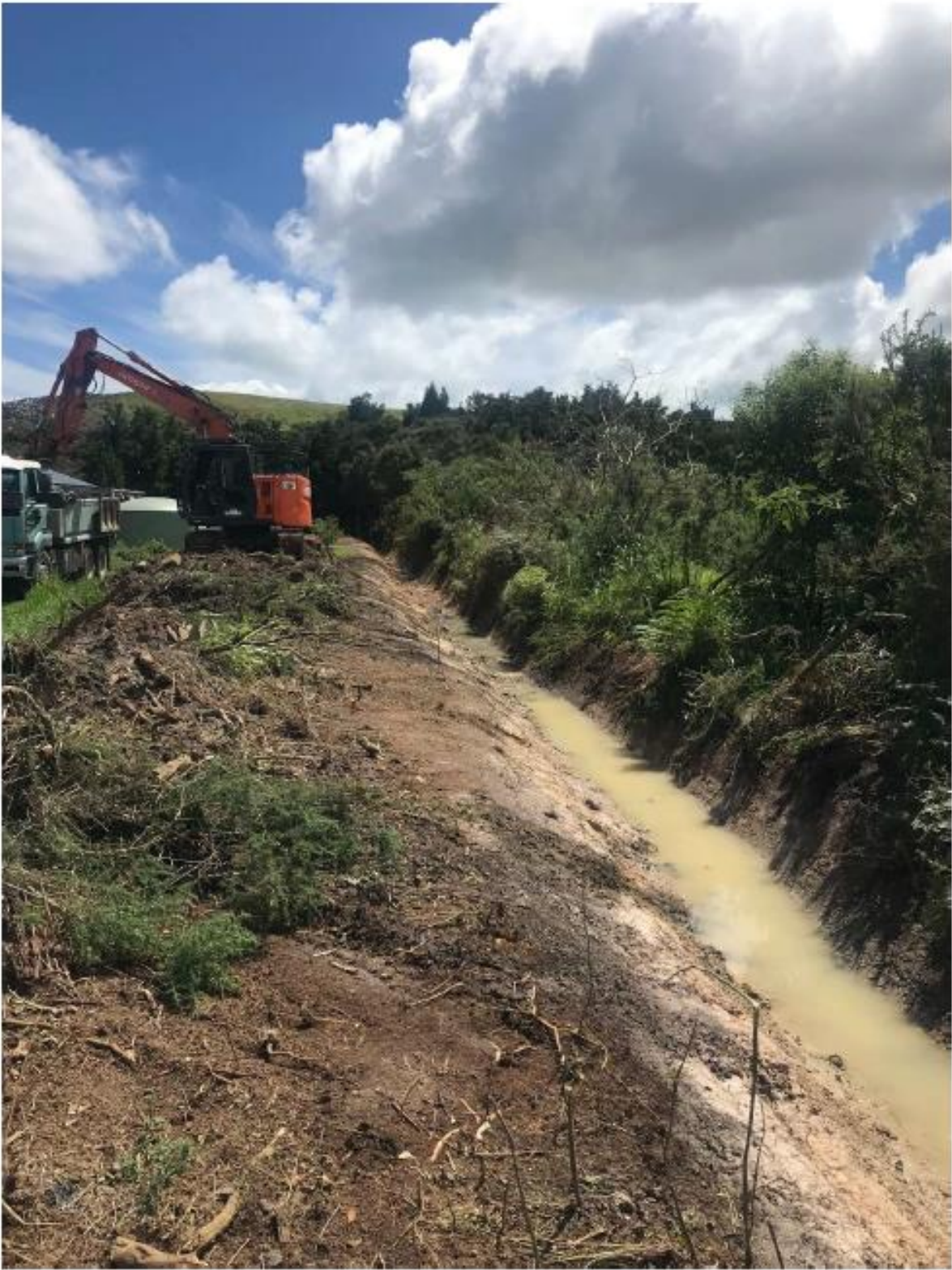
Figure 9: Parapara Toatoa Rd Seal Extension Drainage Works
