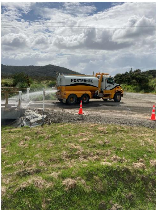
Figure 17: West Coast Rd Bridge Approach
