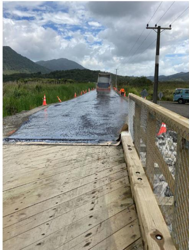
Figure 18: West Coast Rd Bridge Approach
