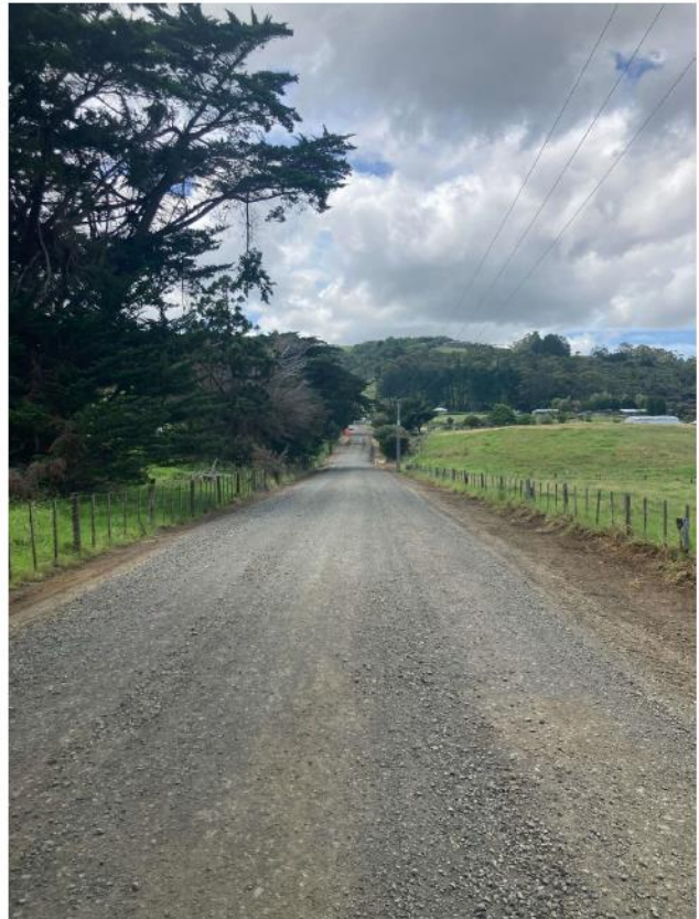
Figure 15: Brass Rd Seal Extension Clearing
