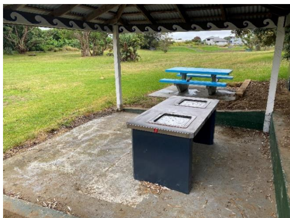
Korora Park BBQ under existing gazebo
