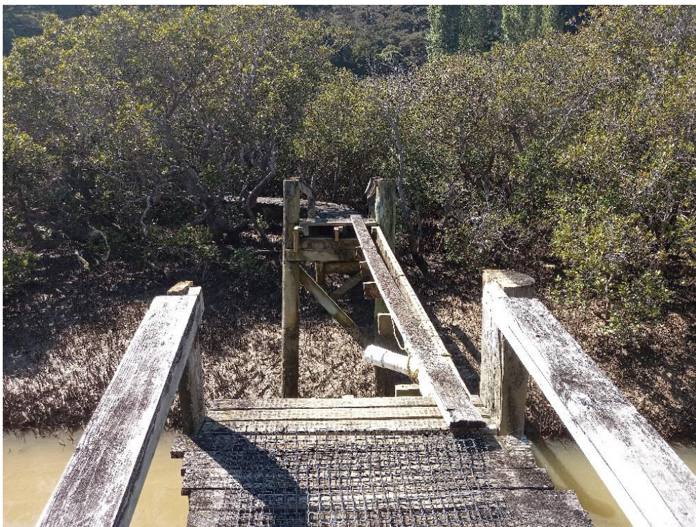
Rotten bridge section of boardwalk removed - Paihia-Opua Walkway
