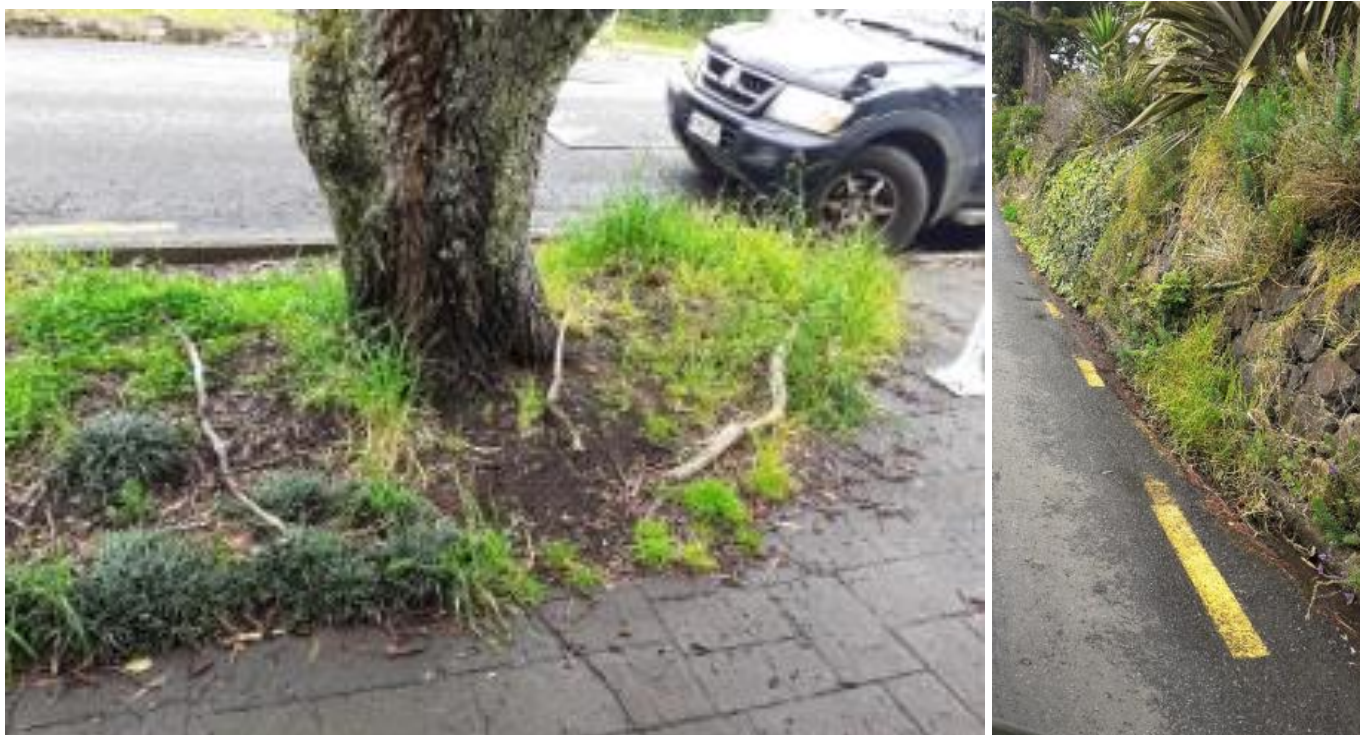
Rawene Township gardens edge control and Clendon Esplanade kerb and channel
