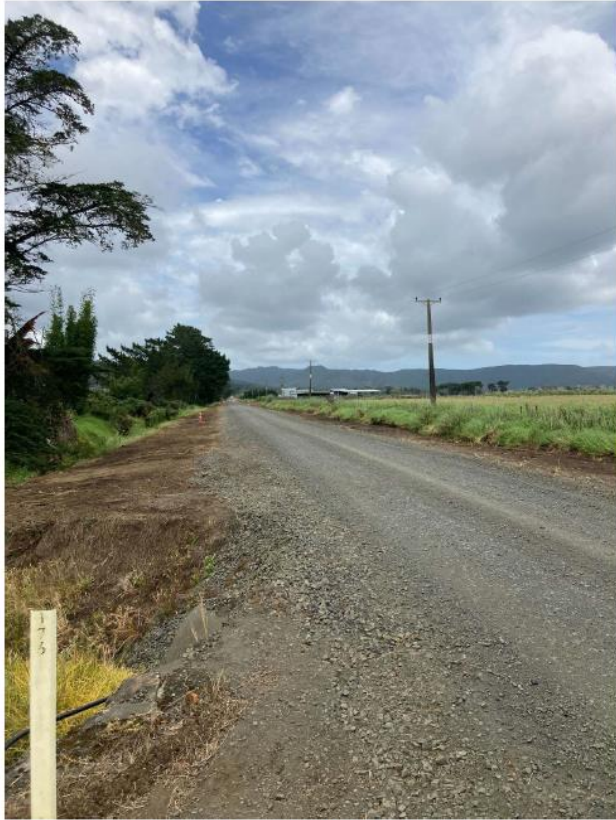
Figure 12: Brass Rd Seal Extension Clearing
