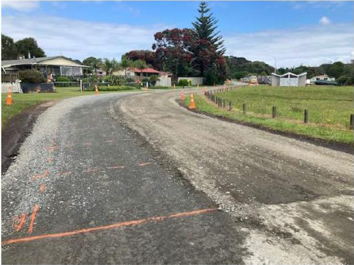
Figure 16: Kaimaumau Rd Seal Extension
