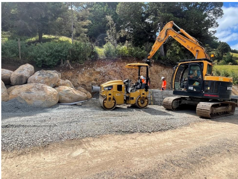
Large rocks waiting to be inspected to confirm relocation
