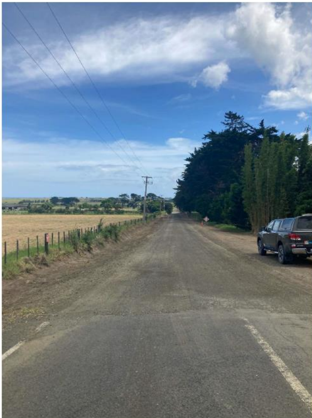
Figure 14: Brass Rd Seal Extension Clearing
