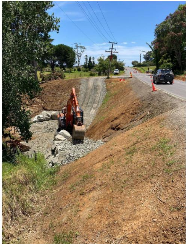
Figure 8: Oruru Rd Rehab 1 Rockwall In Progress
