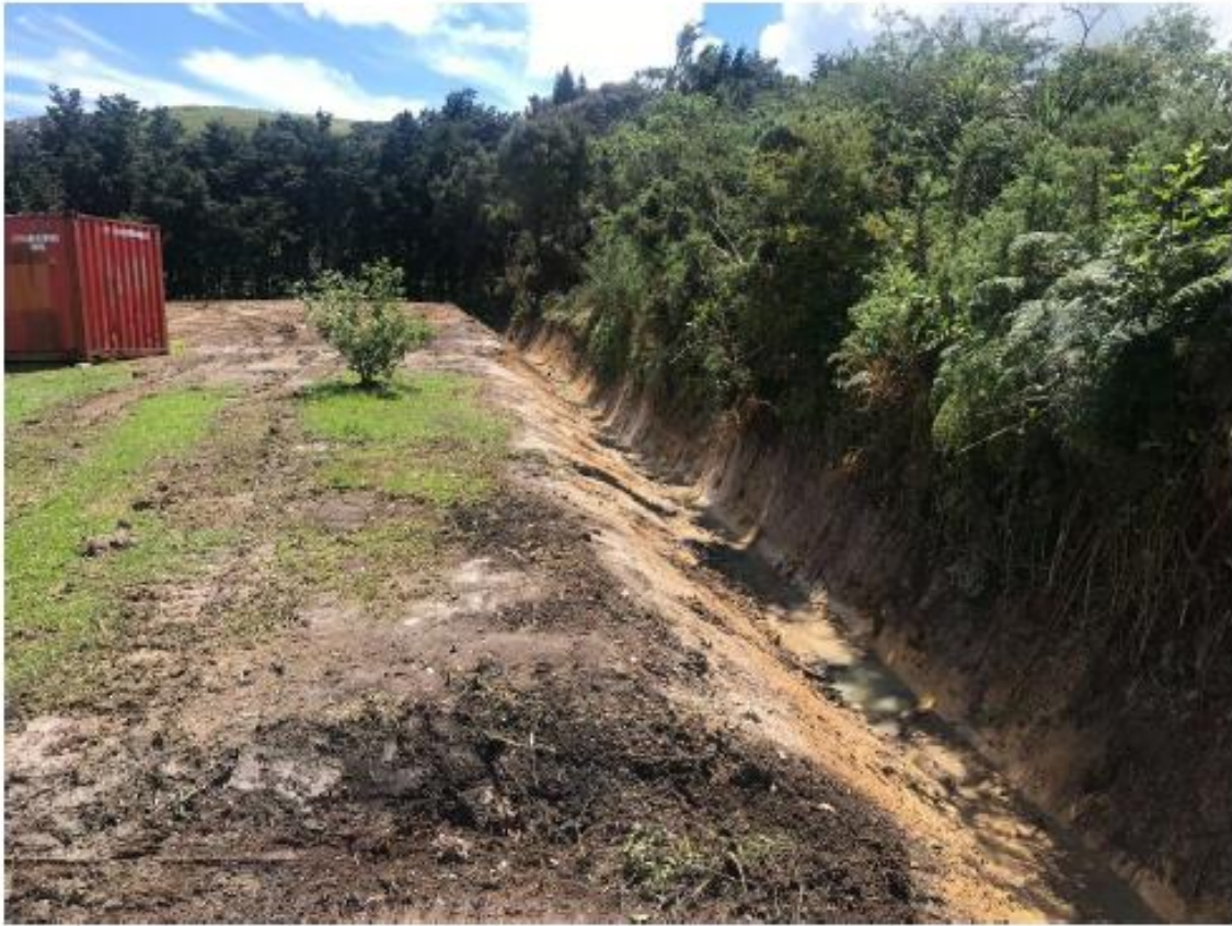
Figure 10: Parapara Toatoa Rd Seal Extension Drainage Works
