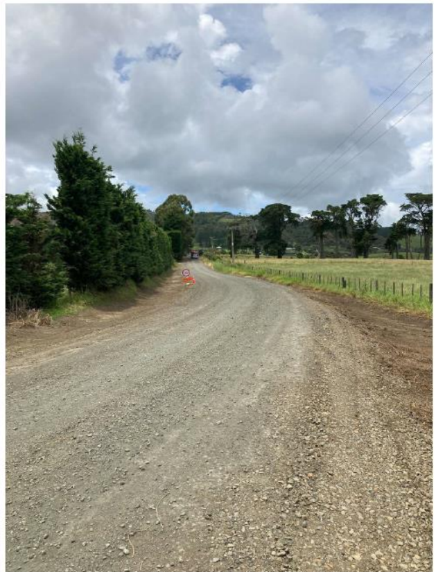
Figure 13: Brass Rd Seal Extension Clearing
