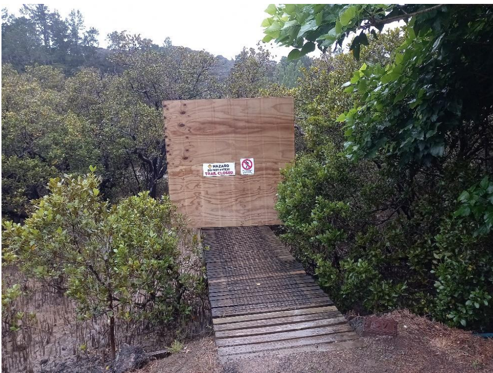
Barriers erected on section of walkway affected by track closure
