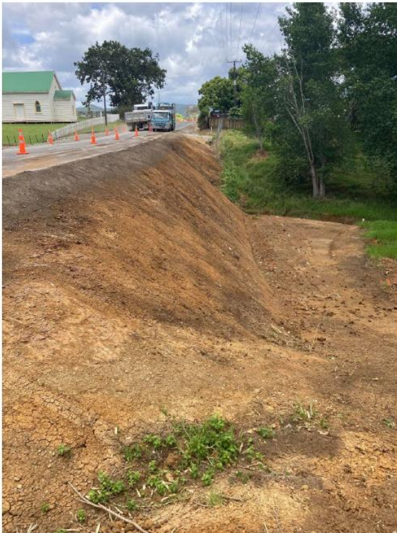
Figure 7: Oruru Rd Rehab 1 Rockwall Preparation
