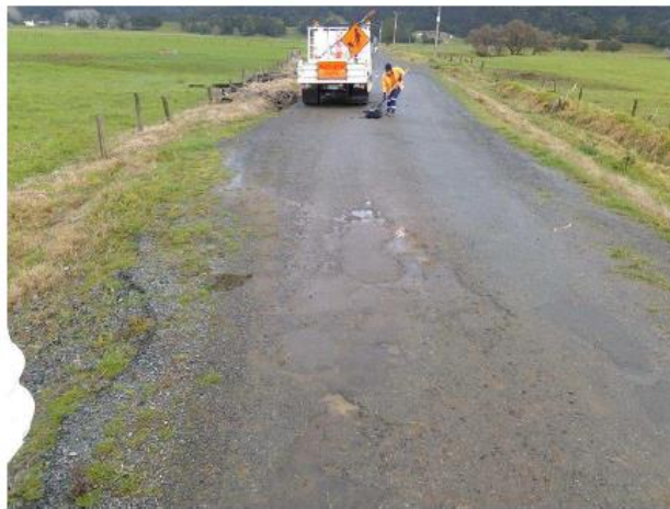
Hariru Rd – Pothole repairs being carried out by Marie & Kahu
