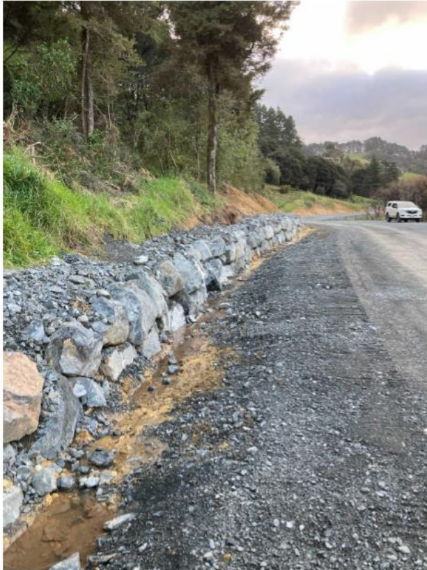
Figure 7: Peria Rd Seal Extension Toe Support
