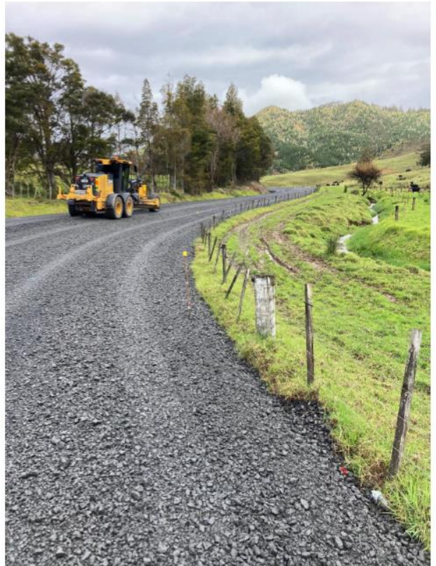
Figure 10: Pawarenga Rd Rehab Pavement Overlay
