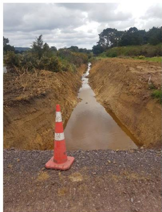
Wahamiti Lane – Outlet Improvements
