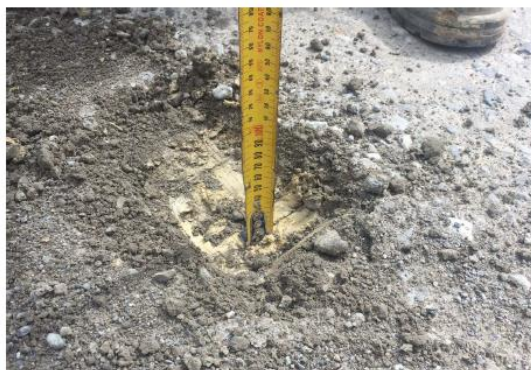
Remuera-Settlement Rd – Test Pit data capturing
