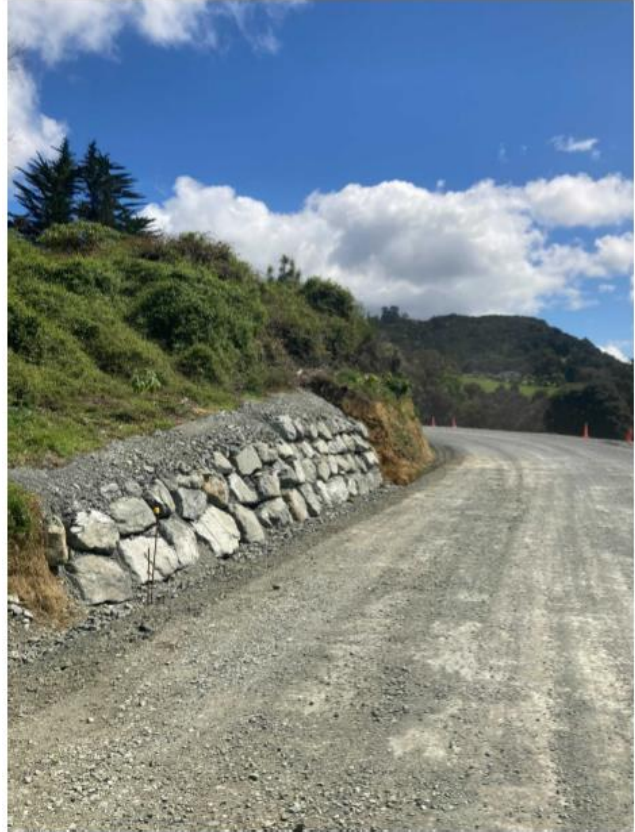
Figure 6: Peria Road Seal Extension Slip Repairs
