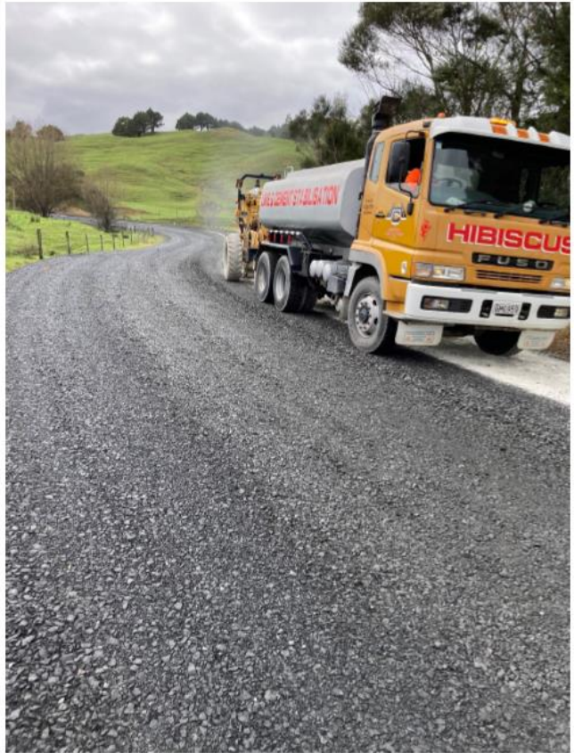
Figure 14: Pawarenga Rd Rehab Stabilising
