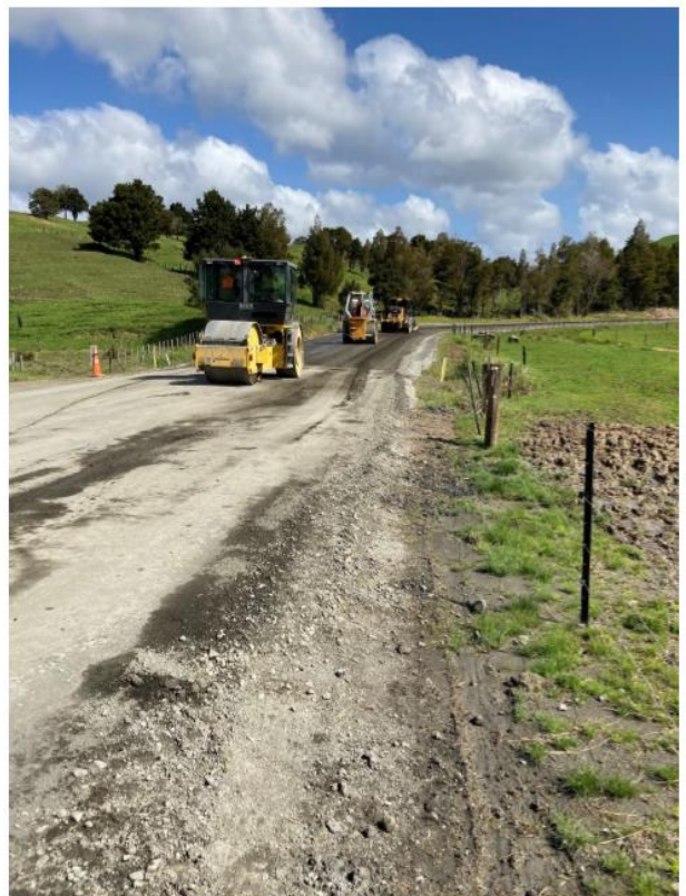
Figure 12: Pawarenga Rd Rehab Stabilising
