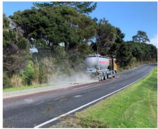
rua - Spread Cement
