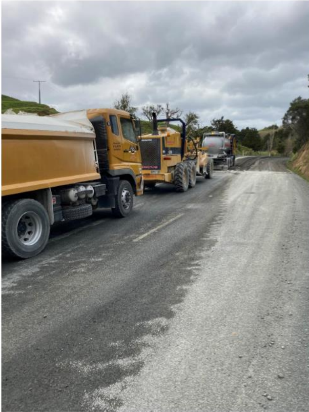
Figure 13: Pawarenga Rd Rehab Stabilising
