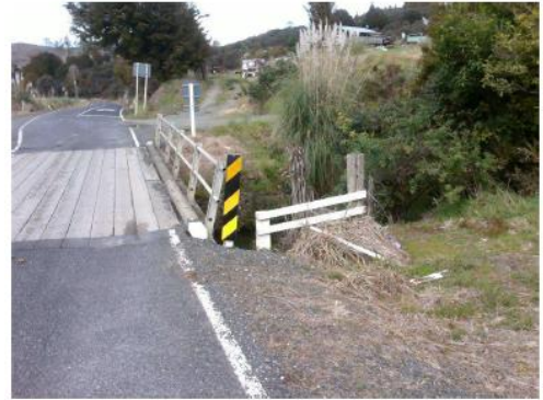
Pipiwai Rd – Missing Bridge End Marker Installed
