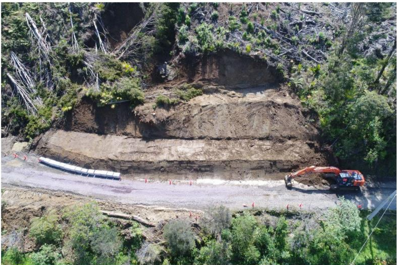
Waimatenui-Mataraua Rd – Slip Retention in progress (Ventia Drone Footage)
