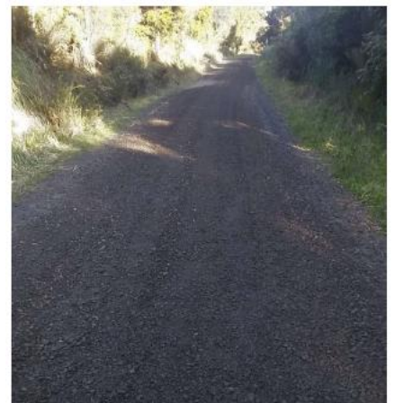
Duddy Rd – Maintenance Metalling
