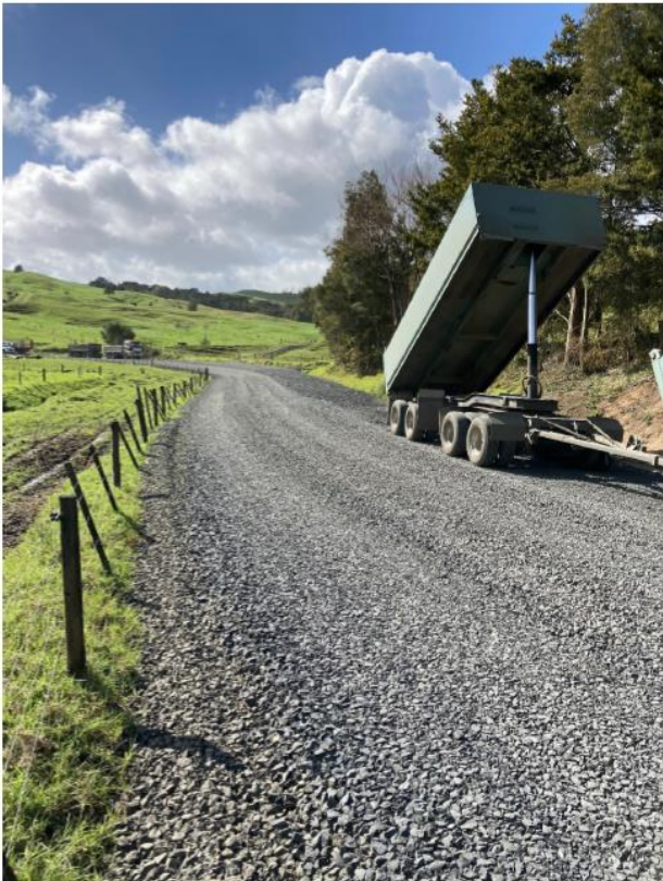
Figure 11: Pawarenga Rd Rehab Pavement Overlay
