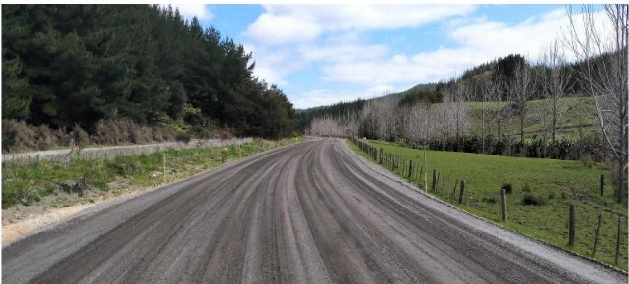
Ngapipito Rd – First 1.6km section slurried up ready for seal
