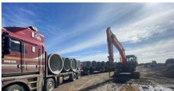
Peras Rd/Wahamati Rd – Culverts being delivered
