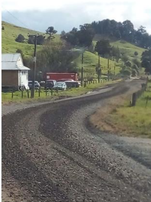
Orakau Rd – Maintenance Metalling
