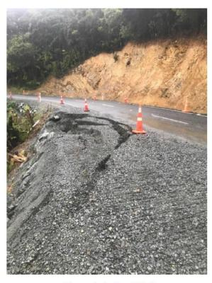
Figure 1: Section Four Underslip
