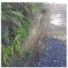
Hupara Rd – Routine culvert end clear with small section of water tabling to ensure adequate drainage.
