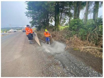
Pungaere Rd – Concrete pumping a new swale in a high discharge area
