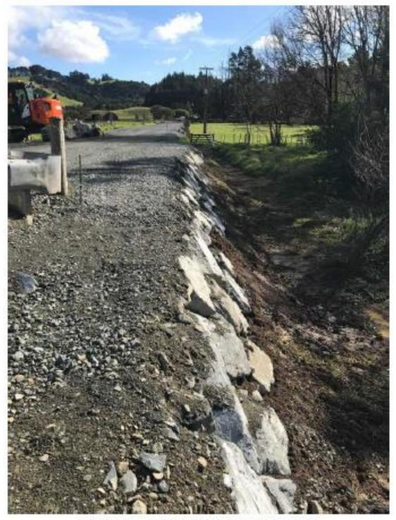
Figure 10: Section 5 Rock wall construction
