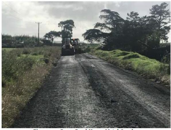
Figure 21: Brass Road Heavy Metal Overlay
