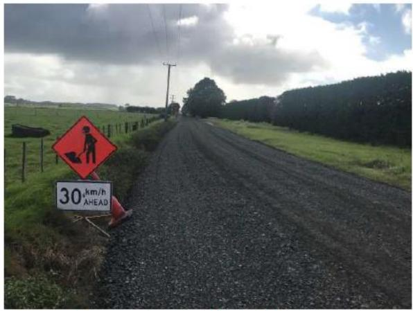
Figure 20: Brass Road Heavy Metal Overlay
