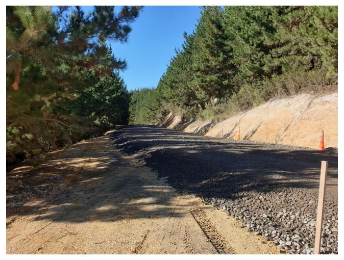
Subbase pavement layer has been overlayed and compacted on Sections 1, 2 and 3 at Ngapipito.
