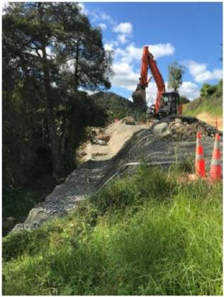
Figure 6: Section 5 Rock wall construction
