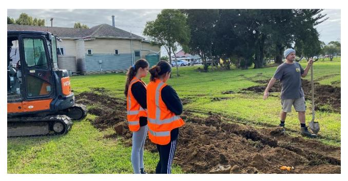
Gateway students getting shown the mega-flow drainage pipe and how it works with the layers of filter cloth, metal and soil by the contractor from Far North Roading doing the sub soil drainage work at Awanui Park.
