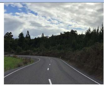
Koropewa Road/ Seal Extension – Pavement ready for sealing
