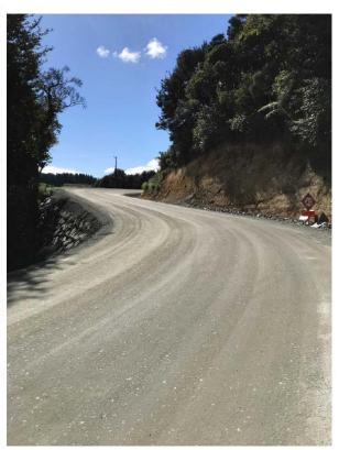
Figure 29: Section Four Ready for seal
