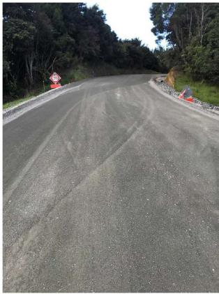
Figure 23: Section Four Seal Prep
