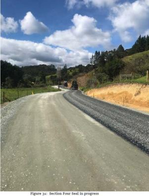
Figure 30: Section Four Seal in progress
