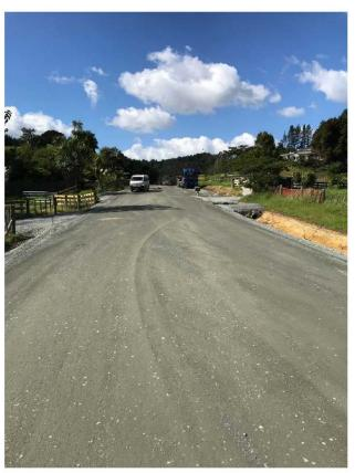
Figure 22: Section Four Drag Brooming
