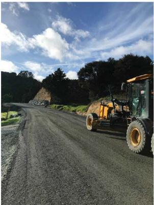
Figure 17: Section Four Seal Prep
