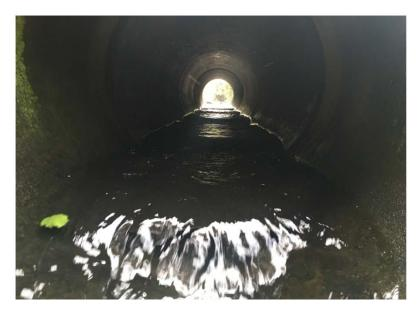
demonstrates the difference in depth, speed and complexity of flow that now occurs inside the pipes. This will assist the upstream migration of native fish. Flexible rubber ramps and mussel rope have also been attached at the culvert outlets to alleviate any perch at low water flows.
