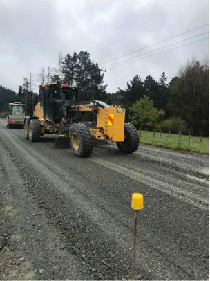
Figure 33: Section Five Pavement overlay
