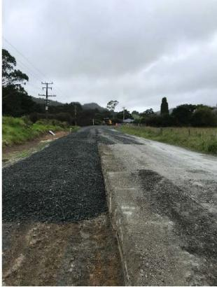
Figure 7: Section Five Pavement undercut
