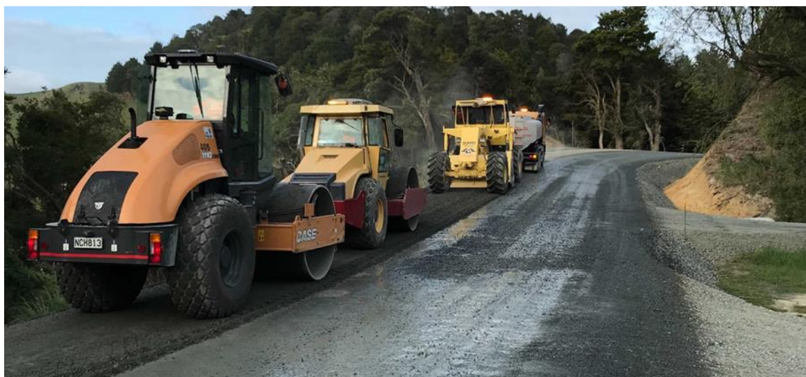
Stabilising in progress at Peria on Section 3
