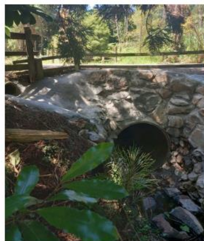
Koranae Rd – Large Concrete Headwall
