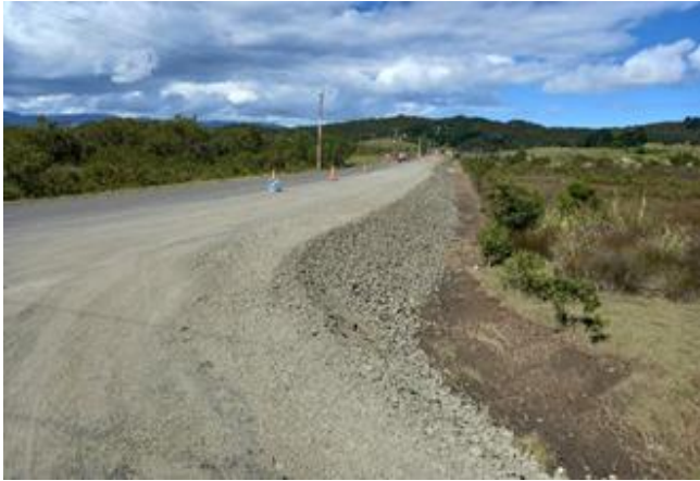
Panguru Road Flood Mitigation/Shoulder Widening
