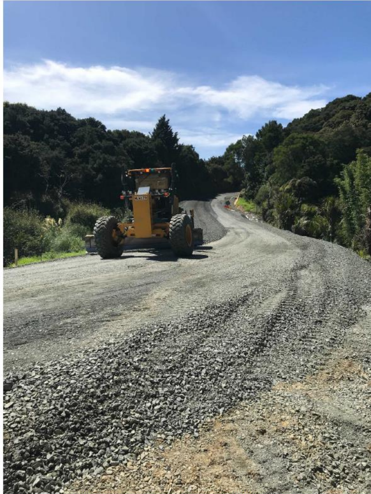
Figure 15: Section Four Overlay in progress
