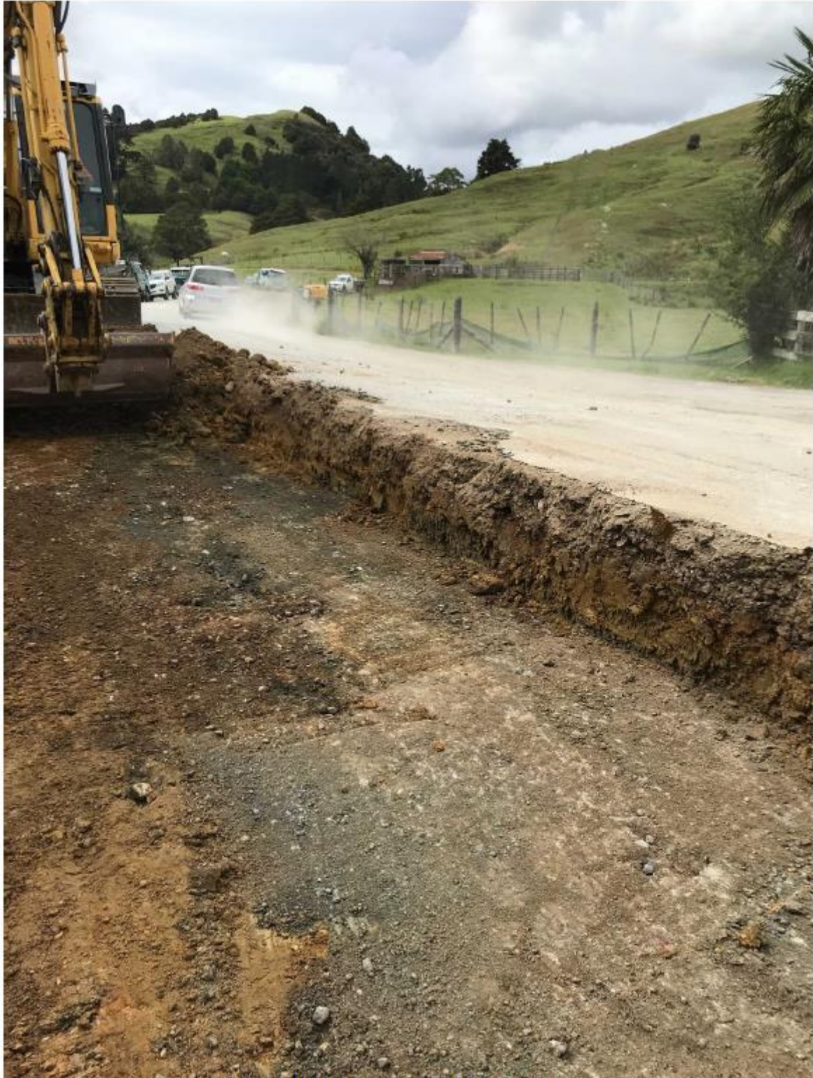
Figure 13: Section Four Bridge Undercut
