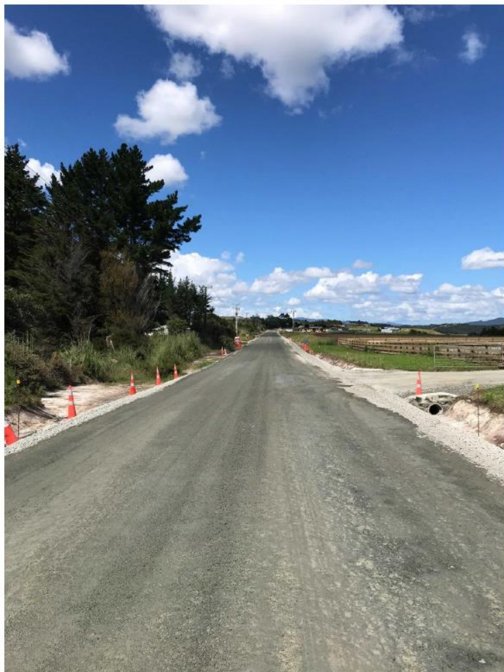
Figure 7: Section One Prepping for seal
