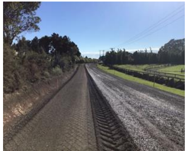
Pungaere Seal Ext. Stabilisation of first 1.4km
