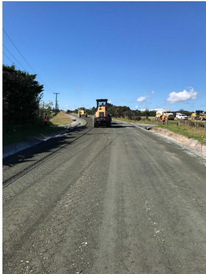
Figure 10: Section Two Stabilising in Progress
