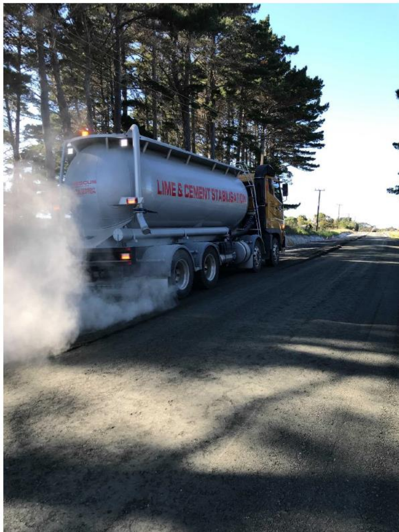
Figure 8: Section Two Stabilising in Progress
