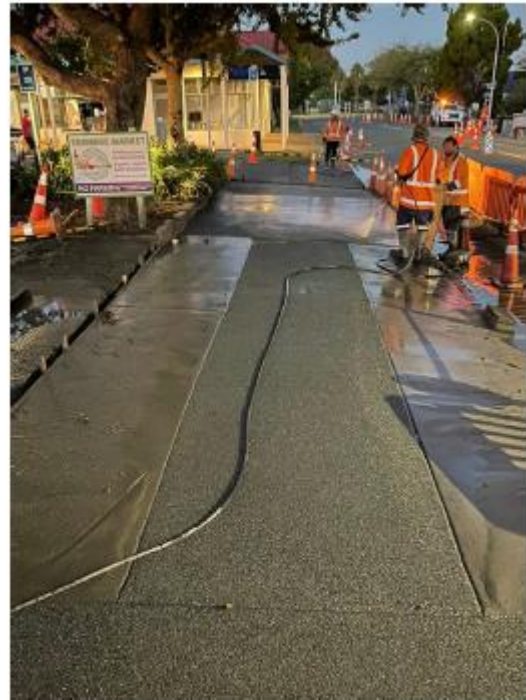
Hobson Ave – Footpath Exposing – Not delineation treatment designed to make it clear for pedestrians where to walk at vehicle crossings.
