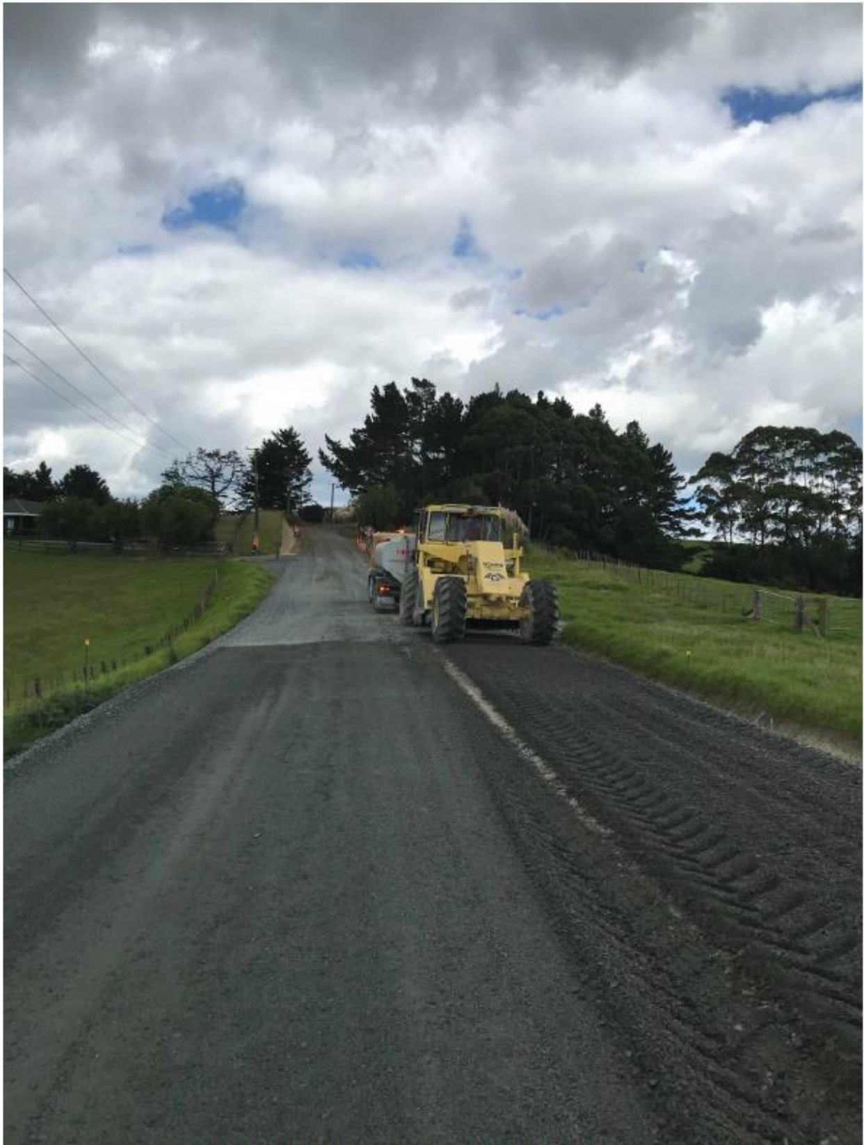
Figure 11: Section Two Stabilising in Progress
