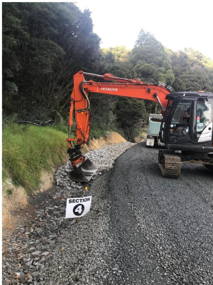
Figure 22: Section Four Scour Protection
