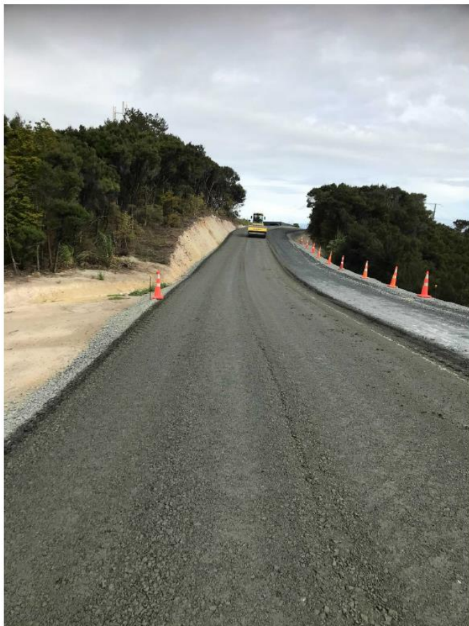
Figure 5: Section One Stabilising in progress
