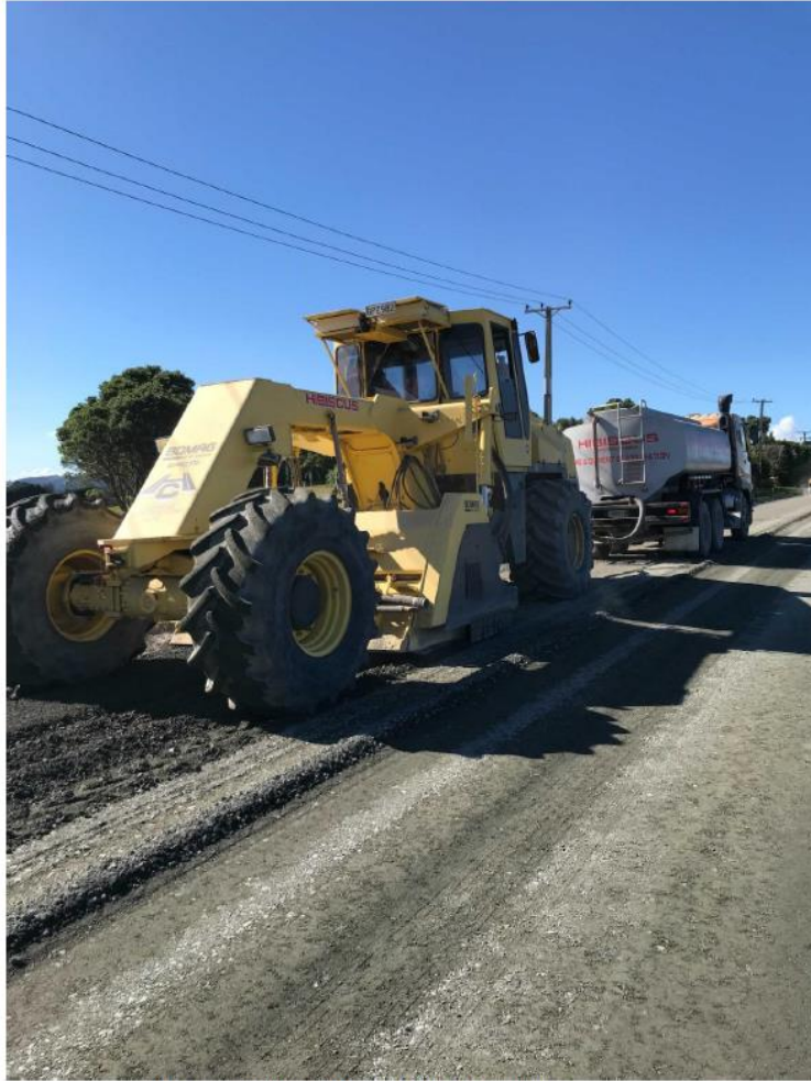
Figure 9: Section Two Stabilising in Progress
