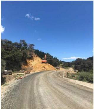
Figure 4: Clearing and corner widening in Section Four
