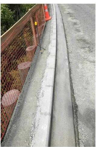
Figure 2: Completed kerb and channel at ch510-575.
