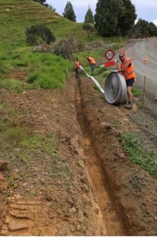
Figure 2: Laying subsoil in water table.
