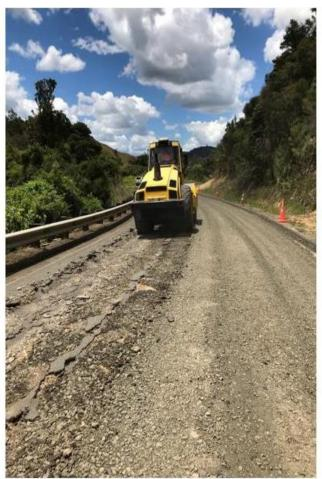
Figure 1: The ripped up pavement being compacted.
