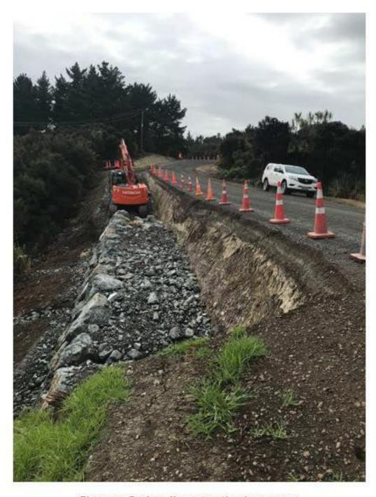
Figure 1: Rock wall construction in progress
