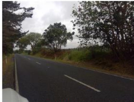
Te Ahu Ahu Road
