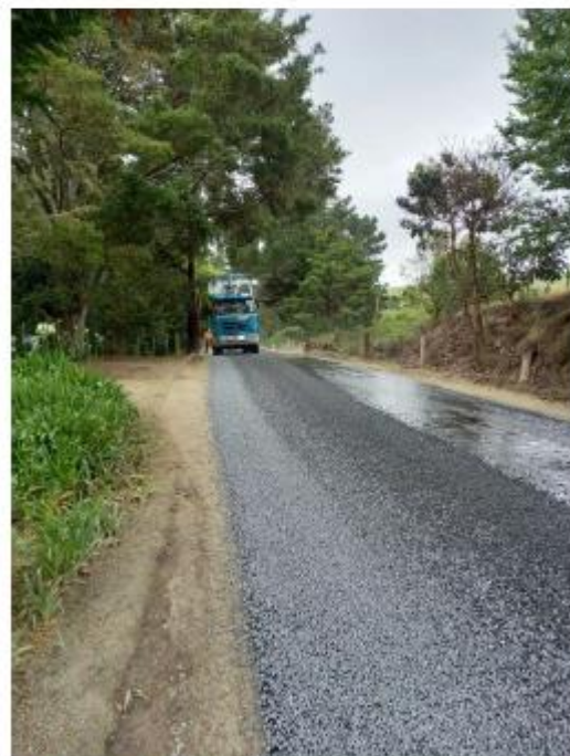
Umarewa School Rd – Dust Sealing site
