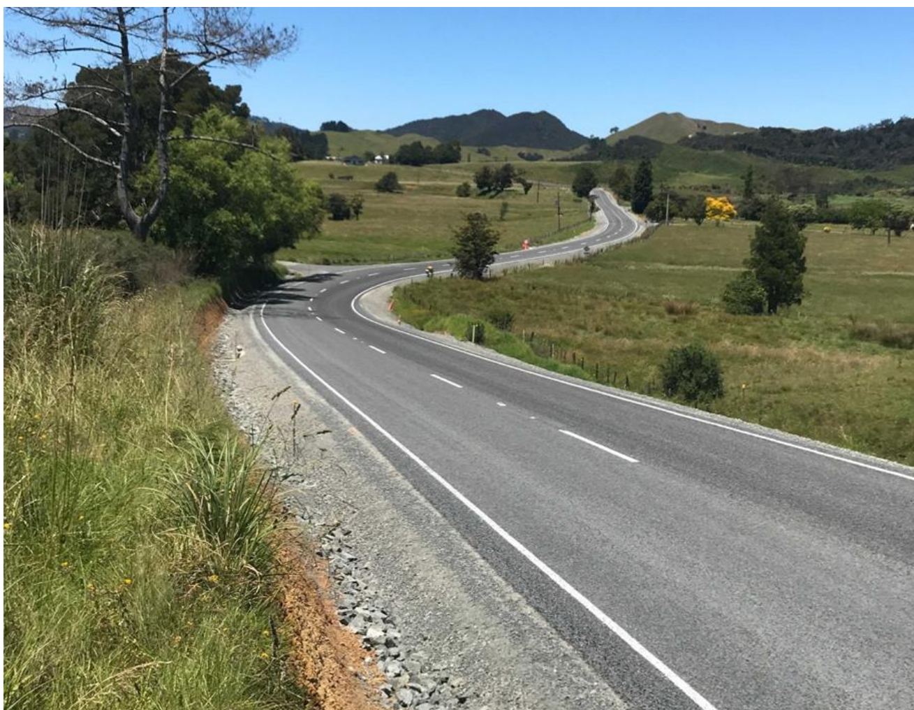
Sealing and linemarking completed at Peria on Section 1
