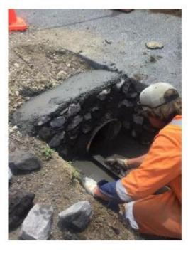
Lance installing a headwall on Blacks Rd
