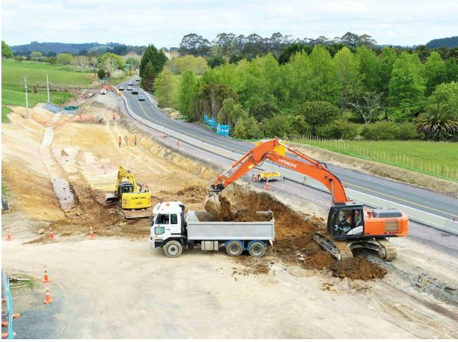
PJ\_utilities: Crew digging a trench to install underground cable for services such as power and fibre. About 2km of services (including stormwater and others) will be installed or relocated across the entire project.
