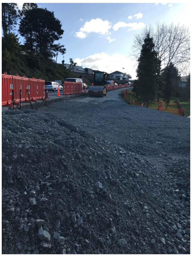
200903\_2: The shoulder being widened to construct the temporary intersection to allow the new intersection to be built. In a few weeks, this will be a traffic lane(s).
