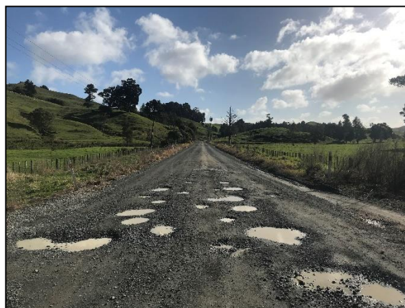
Figure 7.1.2 – Significant Potholing at Bridge Approach
