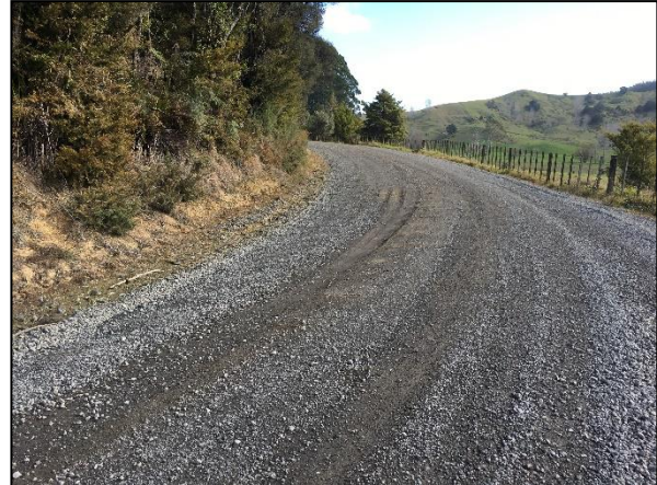
Figure 7.3.2 – Good Superelevation but Limited Drainage
