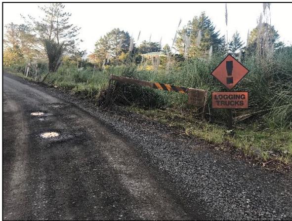
Figure 7.2.1 – Potholing & Logging Signage
