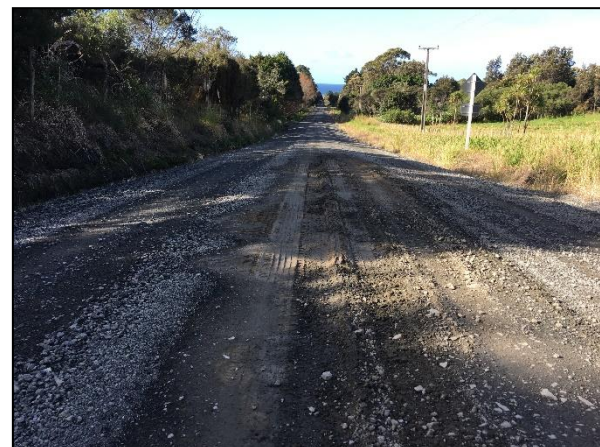
Figure 7.5.4 – Isolated Section of Exposed Subgrade
