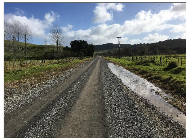
Figure 7.3.4 – Ponding at Carriageway Edge
