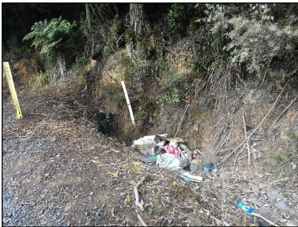
Figure 8.1 – Waikare Road Inlet Blocked with Debris
