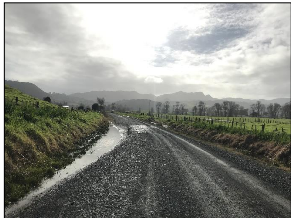
Figure 8.2 – Waimamaku Beach Road Ponding
