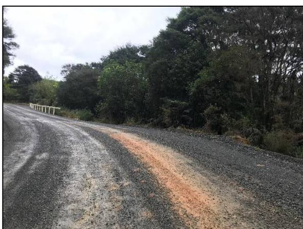
Figure 8.11 – Waikare Road Exposed Subgrade
