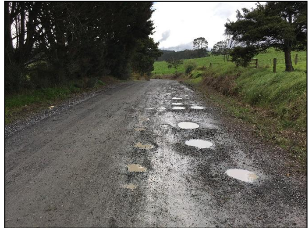
Figure 8.6 – Tapuhi Road with limited crossfall
