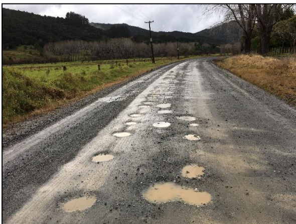
Figure 8.7 – Horeke Road with minimal crossfall
