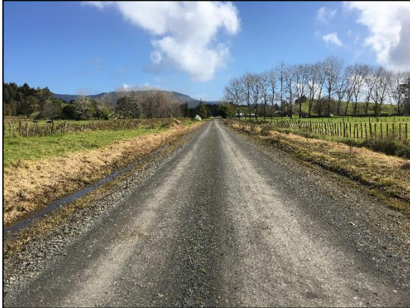
Figure 7.3.1 – Typically Hard Packed Smooth Surface
