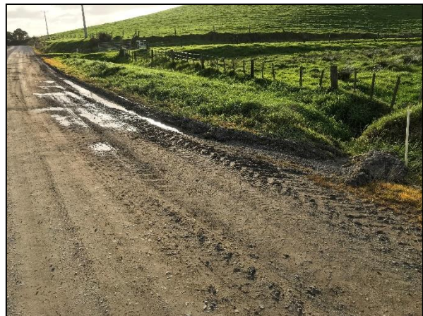
Figure 8.4 – Martin Road Swallow Ineffective Cut-outs
