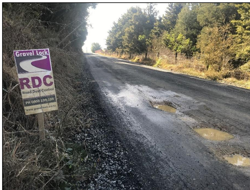
Figure 6.1 – Orakau Road with Gravel Lock RDC section installed
