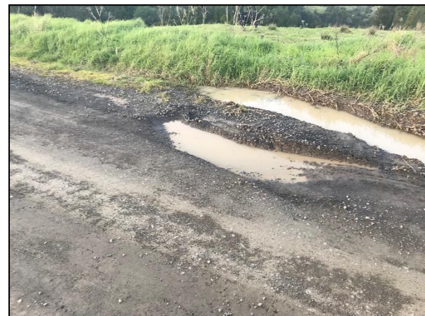
Figure 7.4.4 – Shear Failure at Carriageway Edge
