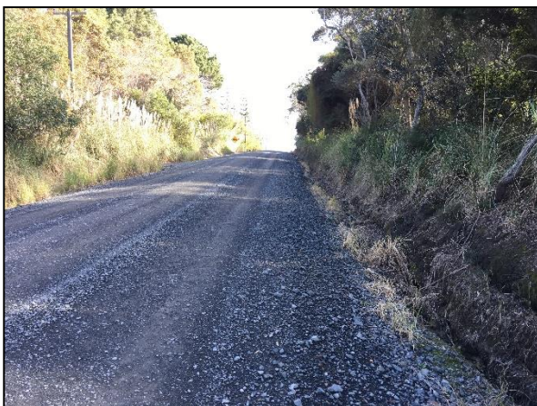
Figure 7.5.3 – Defined Drainage & Crossfall
