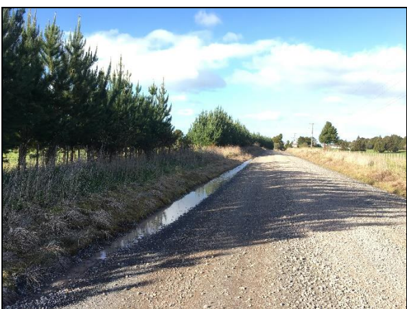
Figure 7.6.3 – Isolated Ponding Through Flats
