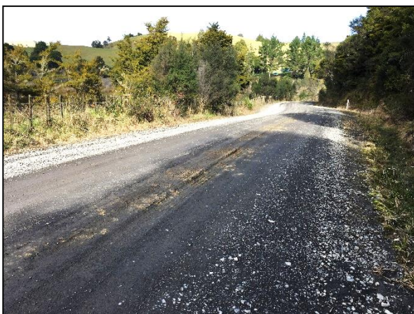
Figure 7.3.3 – Exposed Subgrade
