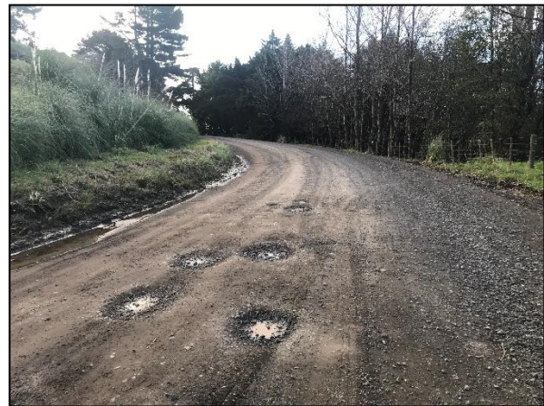
Figure 7.2.2 – Potholing & Ponding on Inside Curve
