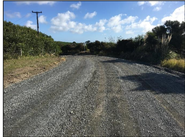
Figure 7.5.2 – Appropriate Superelevation
