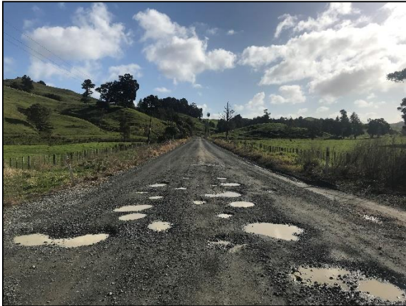
Figure 8.5 – Orakau Road with minimal crossfall
