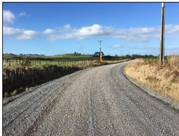
Figure 7.6.2 – Appropriate Superelevation
