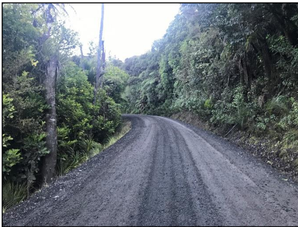
Figure 7.4.1 – Constrained Carriageway – Recent Metal
