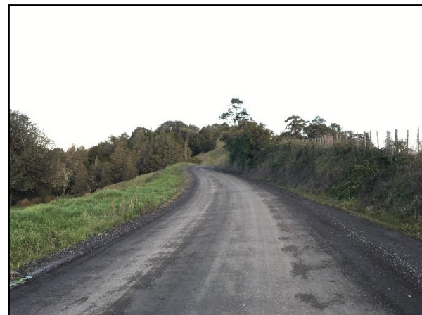
Figure 7.2.4 – Minor Corrugating
