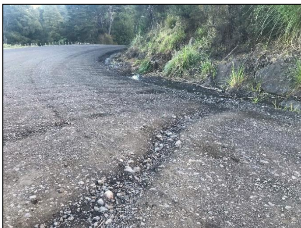
Figure 7.2.3 – Severe Corrugation Causing Scouring
