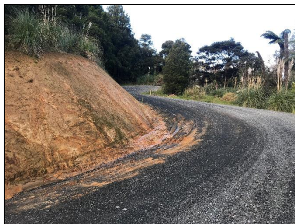
Figure 8.10 – Diggers Valley Road, Exposed Subgrade
