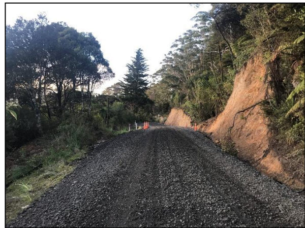
Figure 7.4.2 – Recent Overslip Repair
