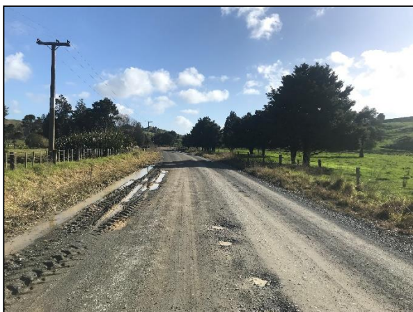
Figure 7.1.1 – Ponding, Shear Failure & Potholing
