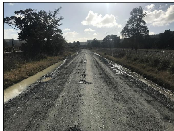
Figure 7.1.4 – Inadequate Drainage
