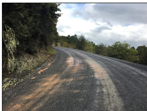
Figure 8.12 – Tapuhi Road Contaminated Running Course
