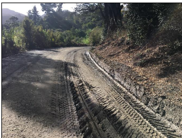
Figure 8.9 – Waitemarama Gorge Road Shear Failure
