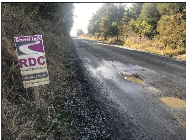
Figure 7.1.3 – Gravel Lock Trial Site Potholing
