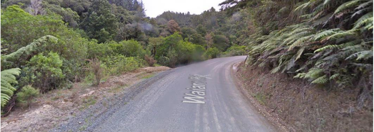
Figure 9: Waiare Road unsealed section proposed 60km/hr speed zone
