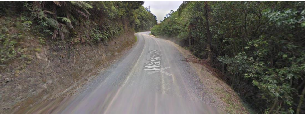
Figure 10: Waiare Road unsealed section showing lack of shoulder areas proposed 60km/h speed zone
