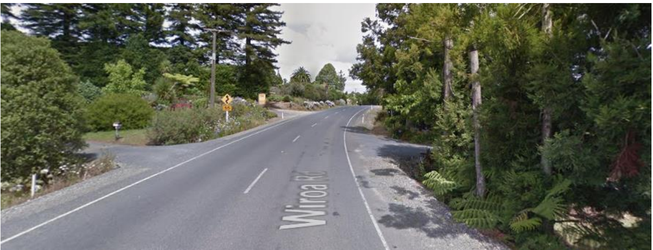
Figure 14: Wiroa Road between State Highway 10 and Waimate North Road
