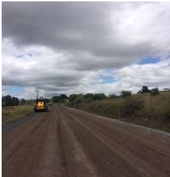
Post stabilisation compaction on Hupara Rd
