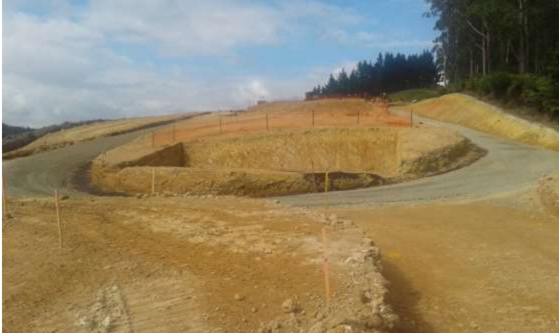
Kerikeri Wastewater Treatment Plant excavation and ring road
