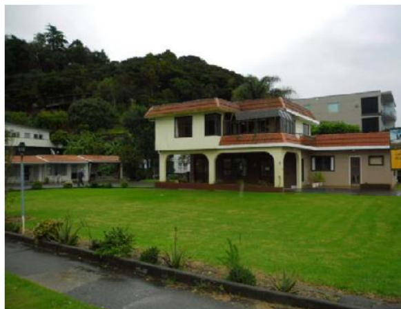
Old motel buildings – demolished October 2013
