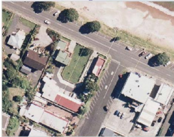
Aerial of the site at the corner of Davis Crescent and 152-154 Marsden Road, Paihia
