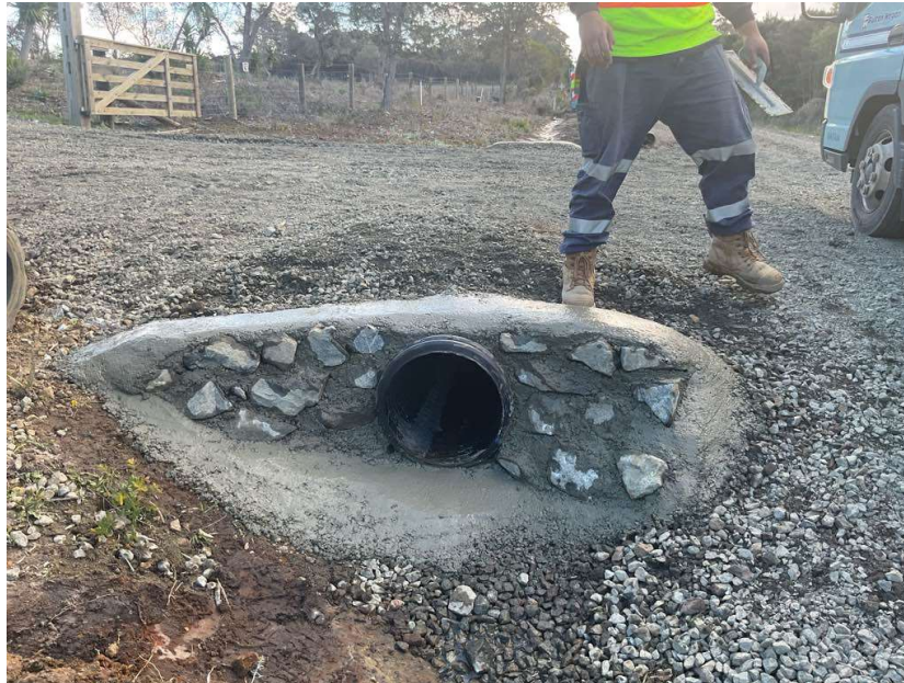
Otaipango Rd – Headwalls
