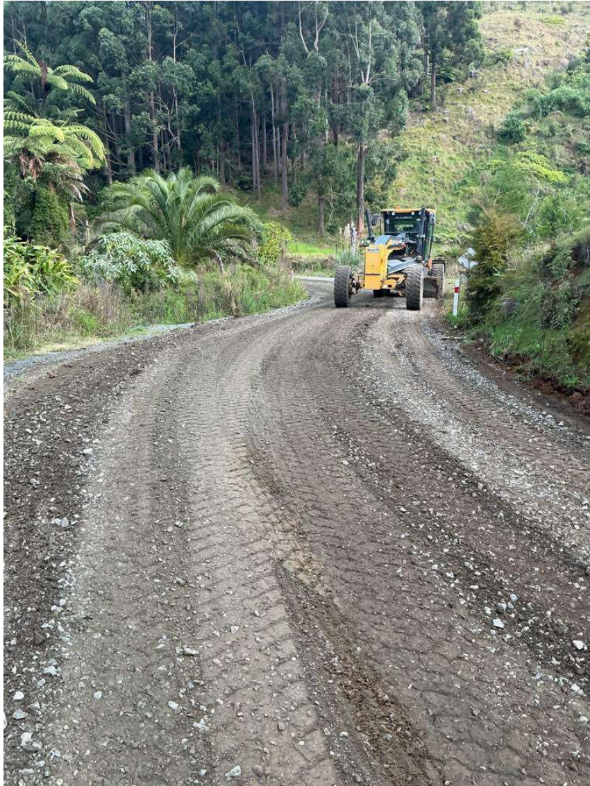
Te Karoa Rd – Maintenance Grading
