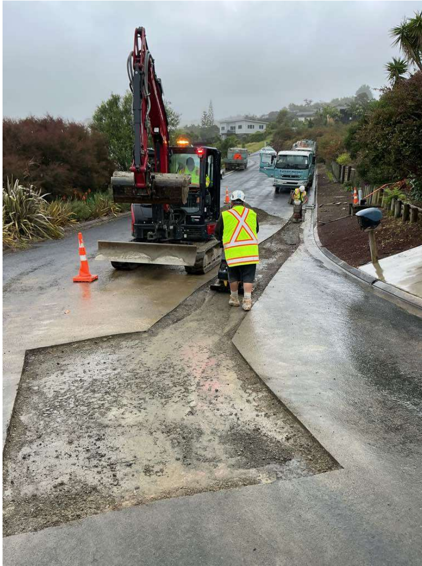
Hibiscus Ave – Sealed Pavement / Drainage Repair
