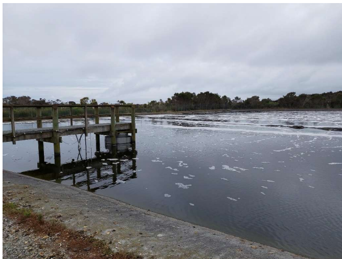
Pond 2 – Looking north across pond 2 at the outlet structure
