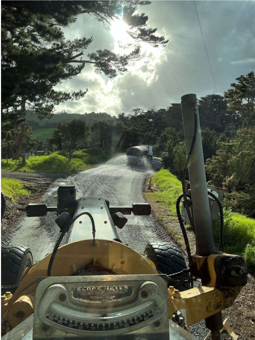
Paponga Rd – Unsealed Overlay in progress
