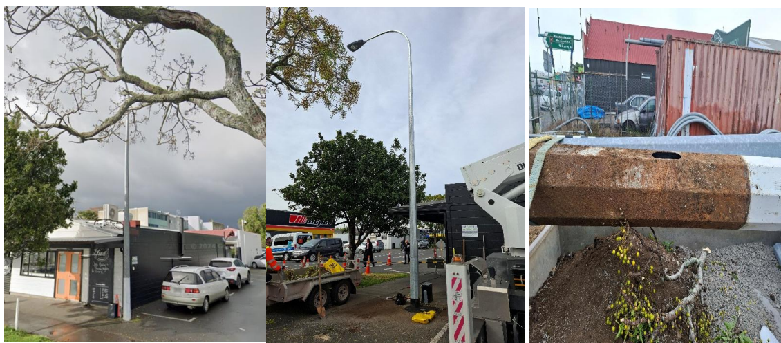
Pole Replacement – Homestead Road, Kerikeri. 31238.
