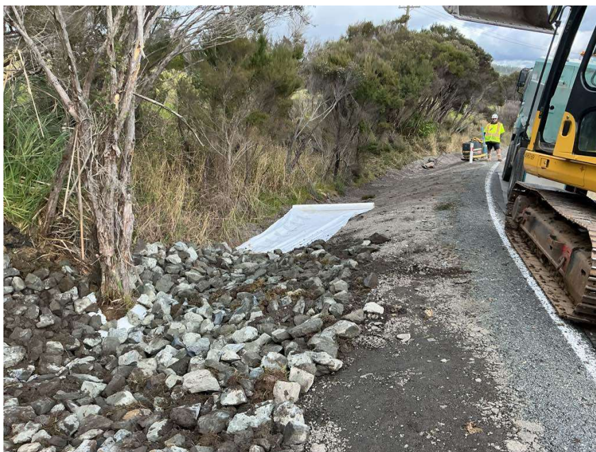
Hihi Rd – Scour Protection / Remediation
