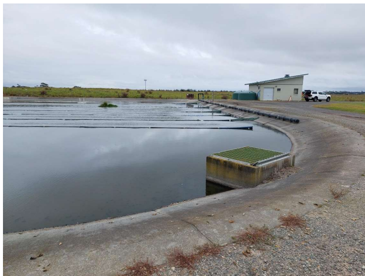
Looking southwest across pond 1 – Outlet structure in the foreground
