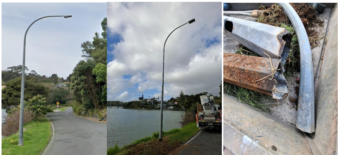
Pole Replacement – Walters Way, Coopers Beach, 32613.
