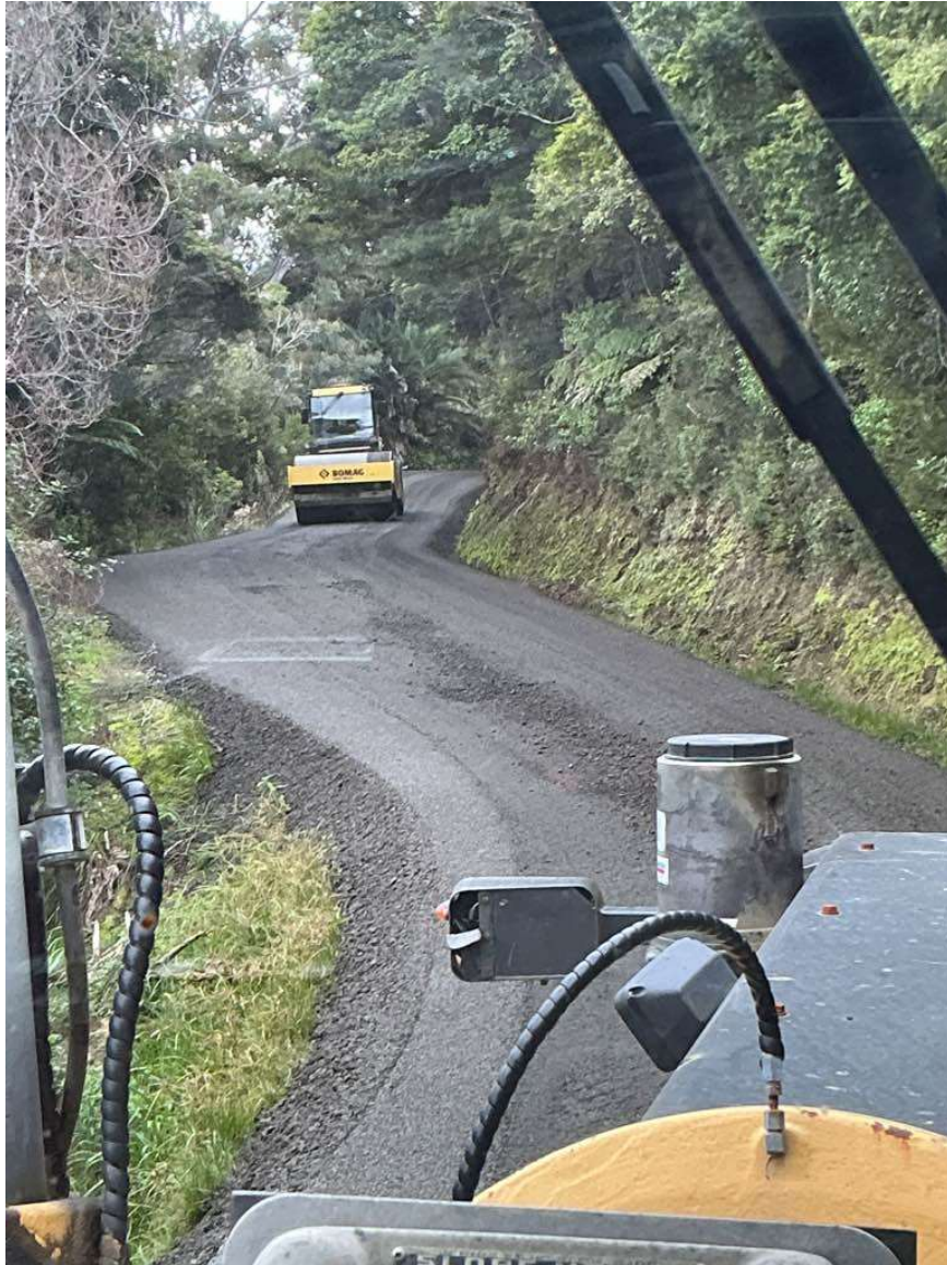
Paponga Rd – Unsealed Overlay in progress
