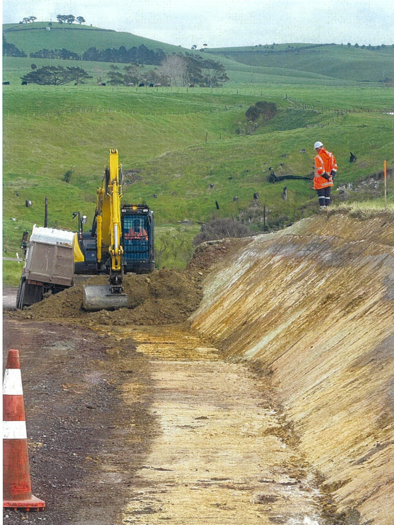
Rangihoua Traction Seal Prep
