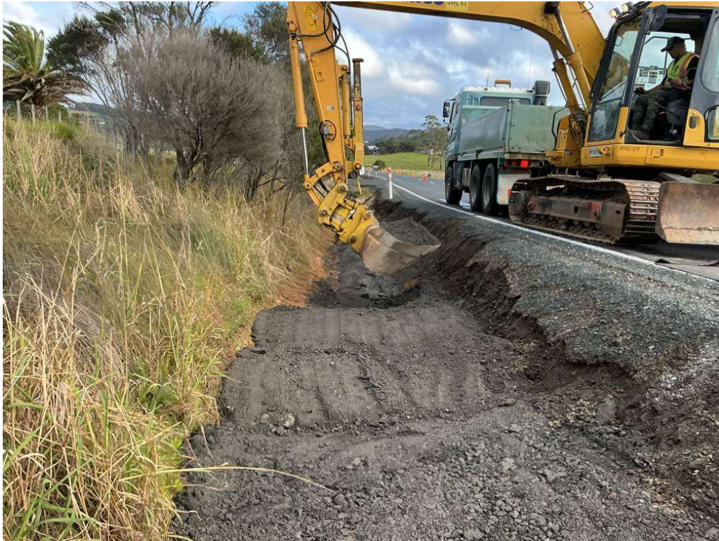
Hihi Rd – Scour Protection / Remediation
