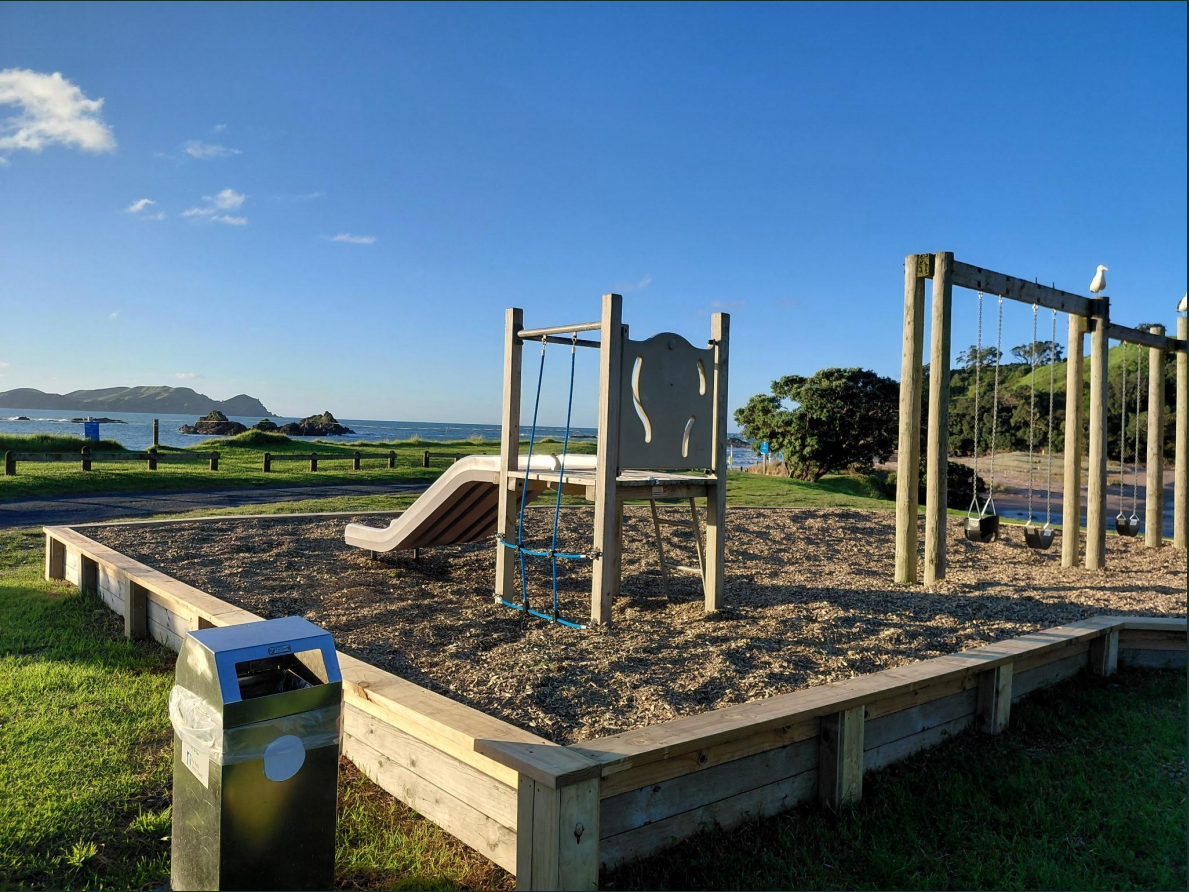
Tauranga Bay Reserve Playground, Tauranga Bay – 36m 3 New retaining wall and capping installed around playground perimeter
