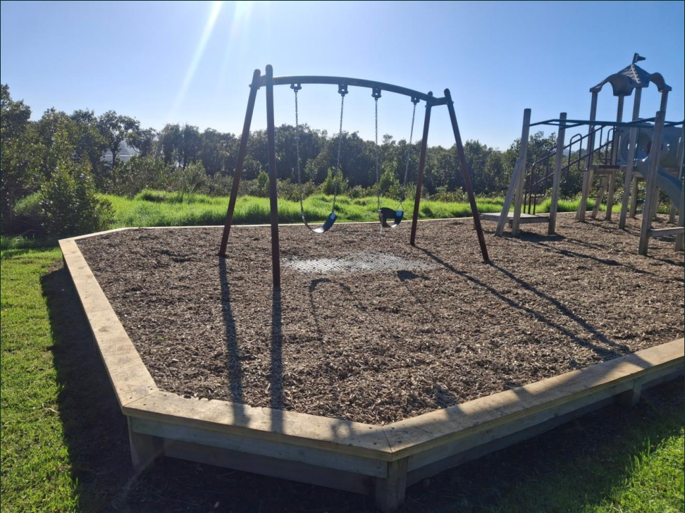
French Reserve Playground, Horeke – 10m 3 New capping installed around retaining wall perimeter
