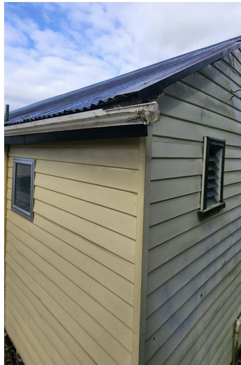
Damaged gutters
