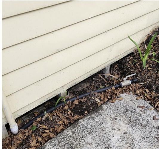
Floor structure touching grade
