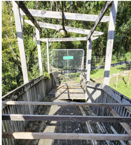
Ramp/deck damage
