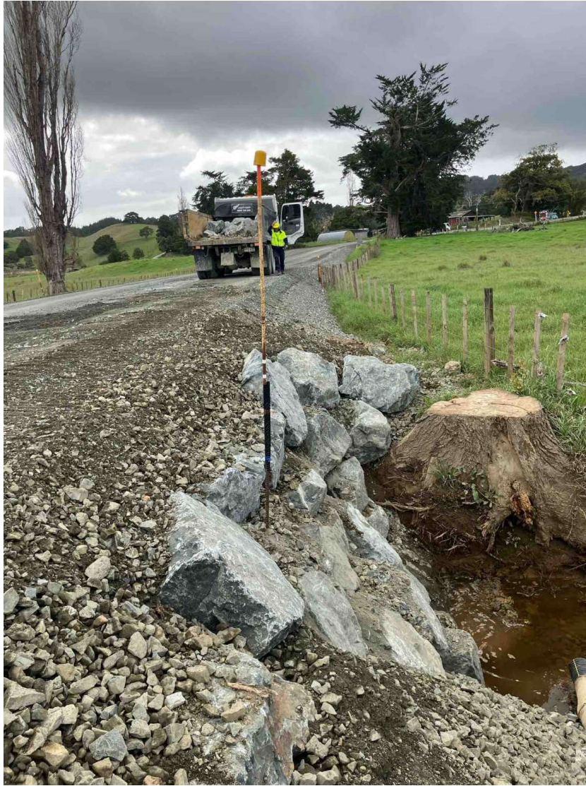
Fairburn Rd Rehab – Culvert headwalls
