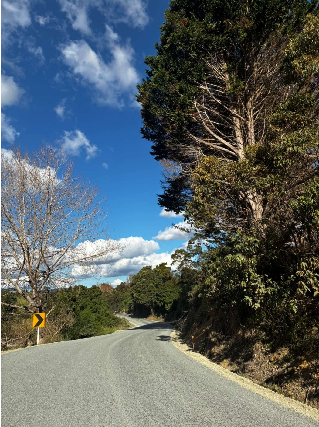
Fairburn Rd Rehab – New Seal
