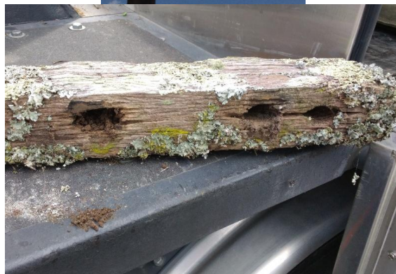
Paihia & Kawakawa, light replacements – 31792, 31794
