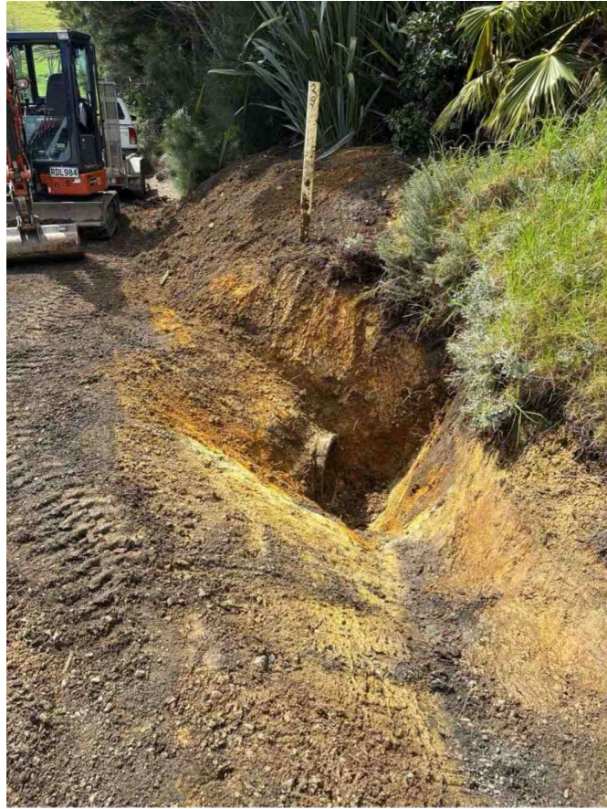
Oinu Rd – Culvert end clearing
