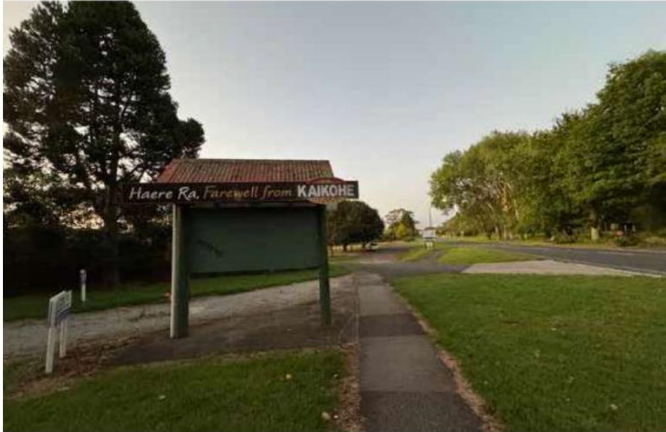
Looking south-west along state highway 12, with existing signage and pull over area in the distance. Cycle trail track to the left of image.
