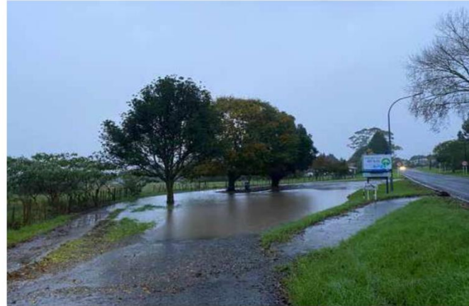
Looking south-west along state highway 12, flooding evident in pull-over area
