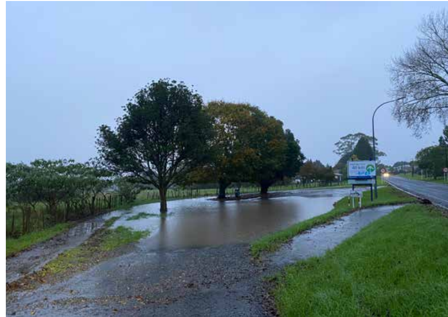
Looking south-west along state highway 12, flooding evident in pull-over area
