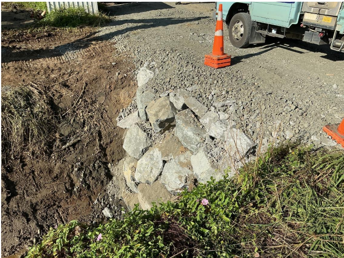
Wells Road Drainage Renewals – Complete
