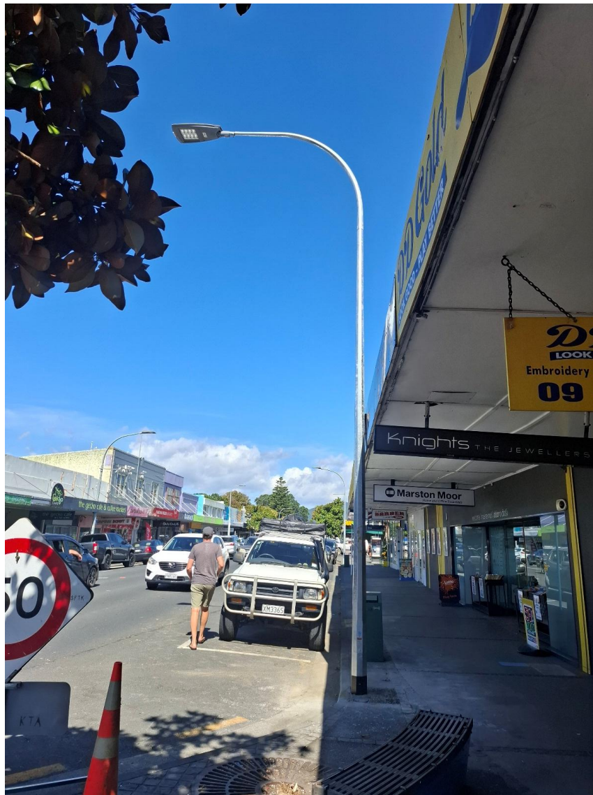
30831 Omapere Rd, Kaikohe – Pole replacement.
