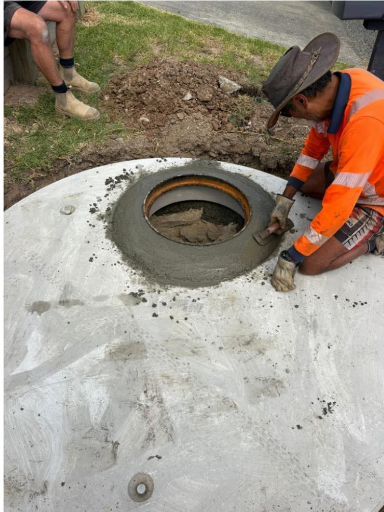
Ocean View Rd – Drainage upgrade in progress (Sweetwater Construction)
