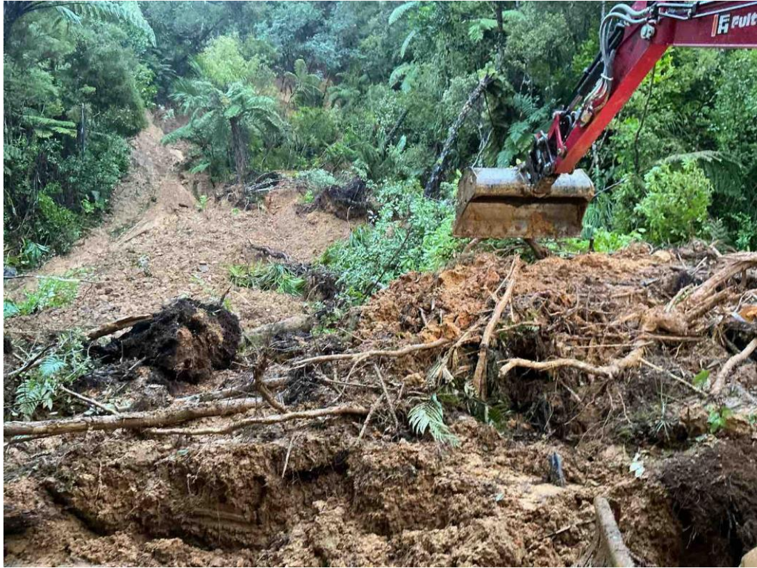
Takahue Rd – Overslip clearing in progress
