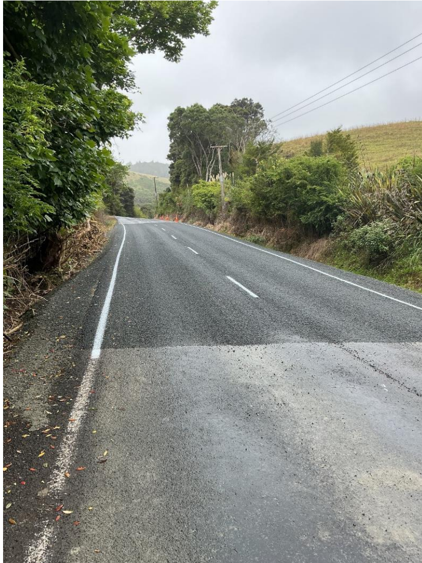
Totara North Rd – Subsidence Pavement Repair Completed
