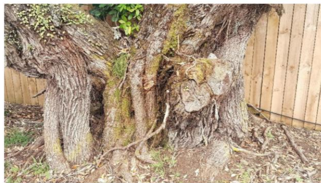
Figure 5: Showing the size of this large decay ingress.
