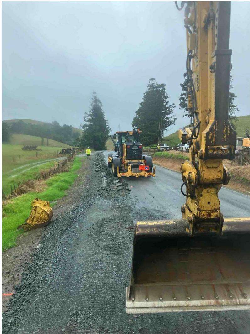
Fairburn Rd Rehab – Shoulder undercuts in progress
