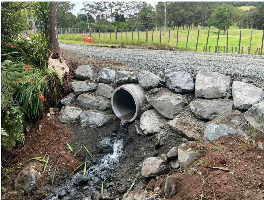
Kaiawe Rd – Culvert Replacement
