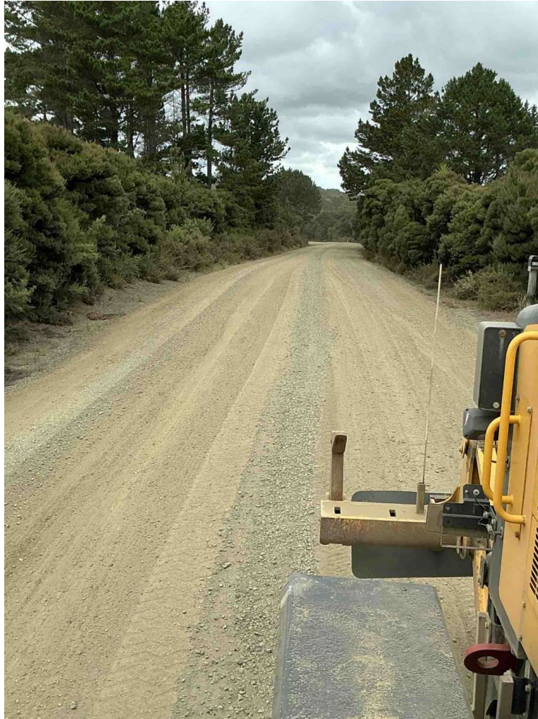
Te Hapua Rd – Maintenance Grading in progress
