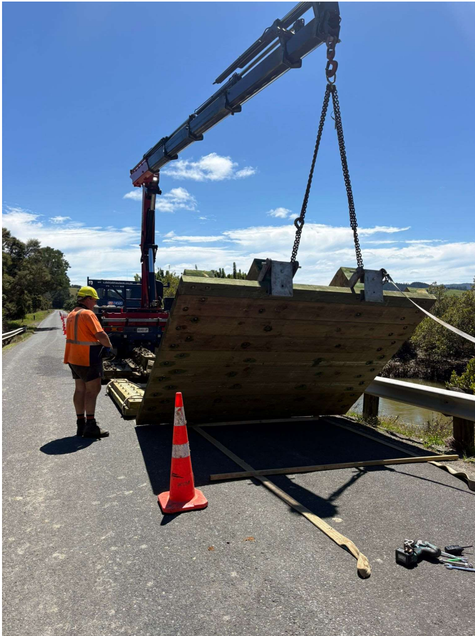
Kohukohu Rd Floodgate Repair
