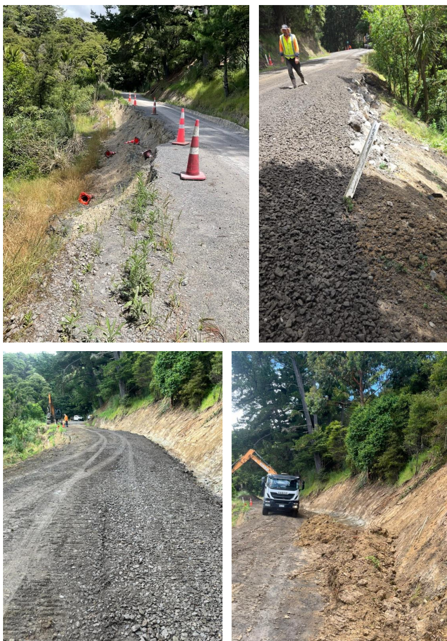
Taheke Road – Underslip Repair / Widening
