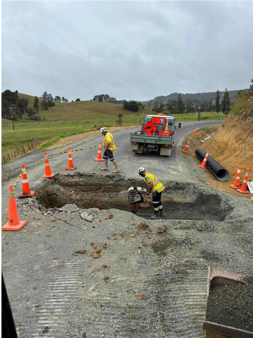
Fairburn Rd Rehab – Drainage replacement in progress
