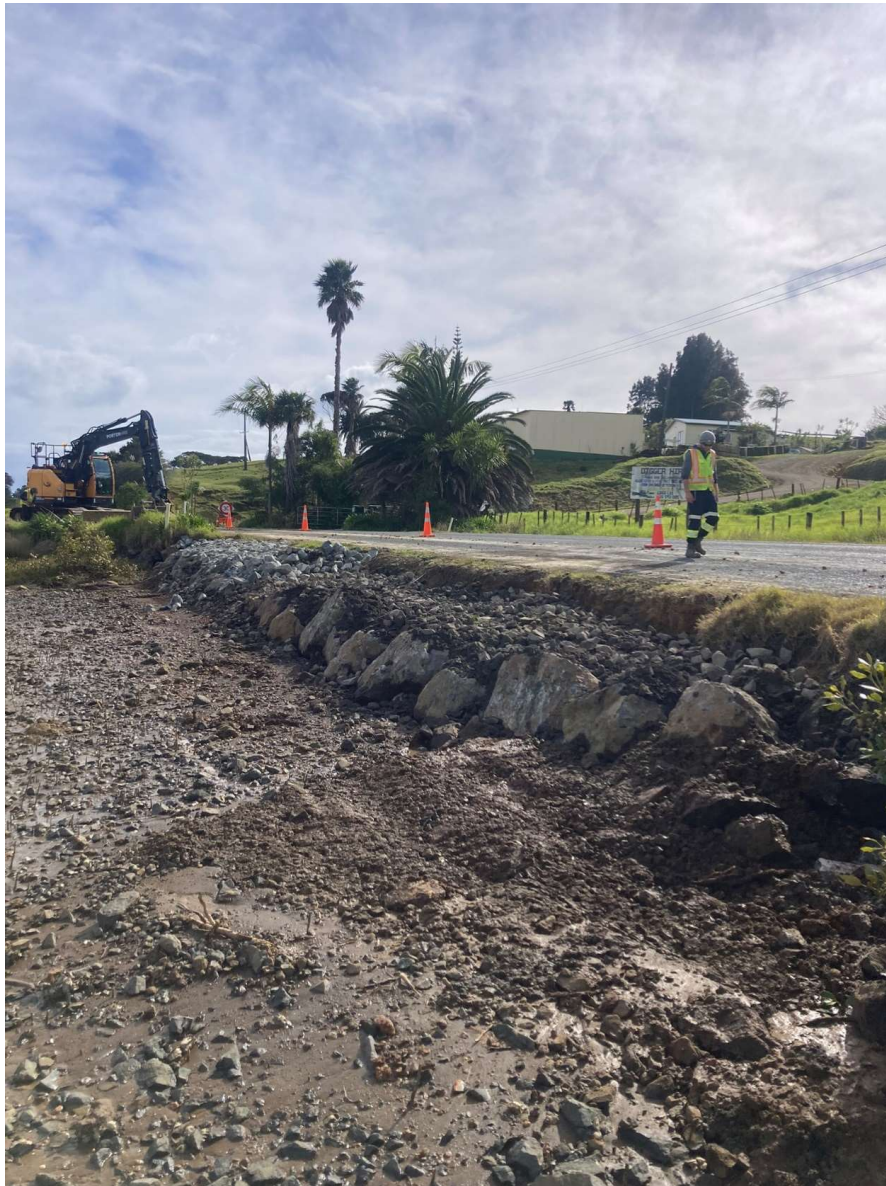
Hihi Rd – Rock Wall Repair in Progress
