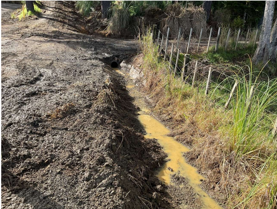
Yuretich Rd – Culvert End Clearing
