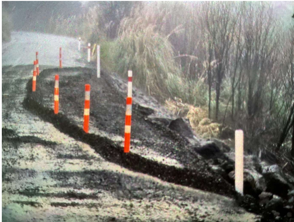
Paranui Rd – Bund and delineate Underslip
