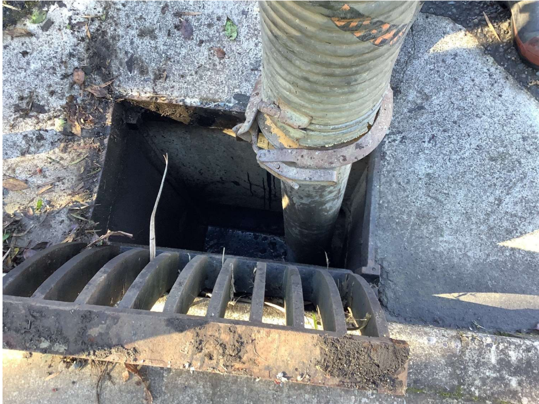
Bank St, Kaitia – Cesspit chamber clearing
