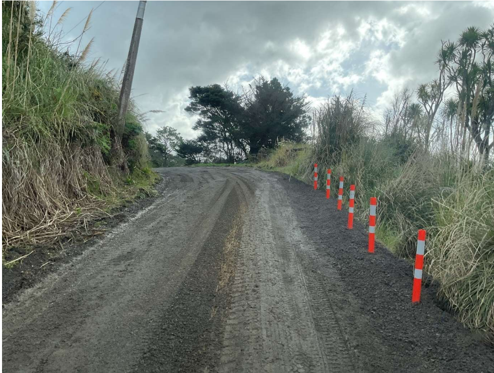
Rangi Point Rd – Bund and Hit sticks around Underslip
