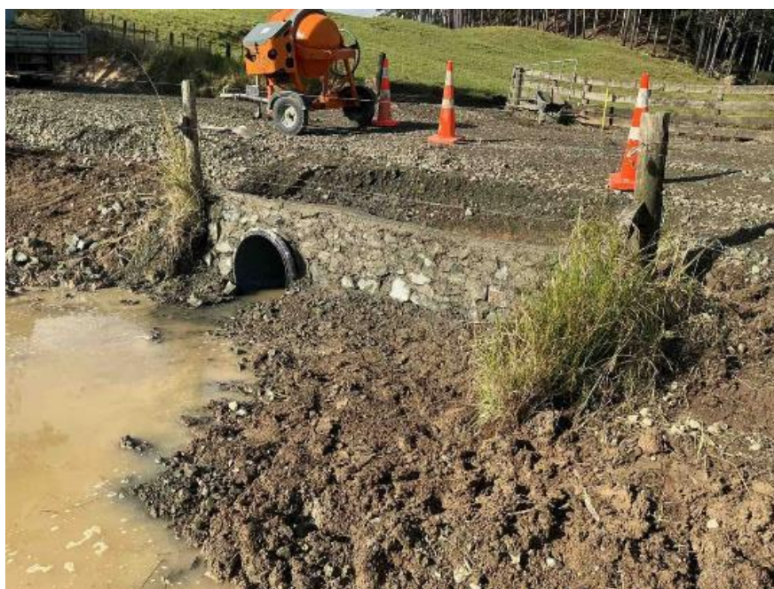
Peria Valley Rd, Kaitaia – Culvert Headwall
