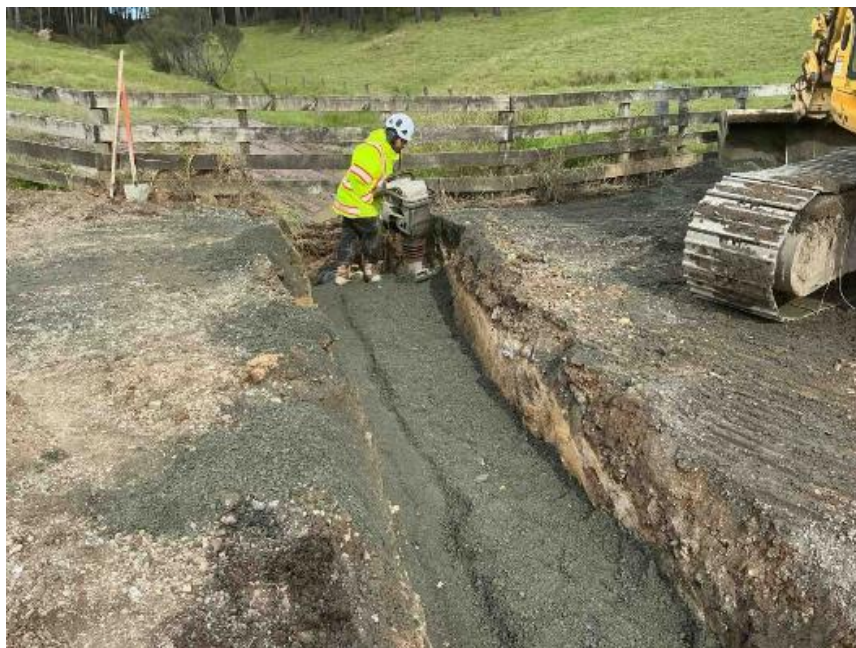
Peria Valley Rd, Kaitaia – Culvert Replacement In Progress
