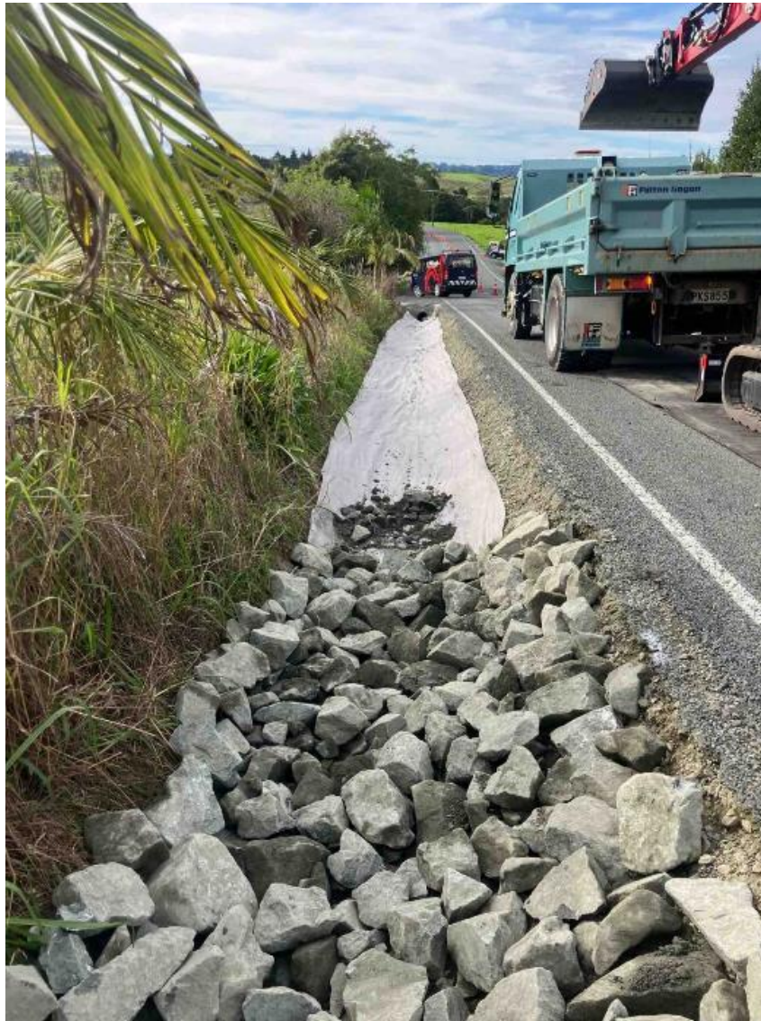
Larmer Rd Rehab – Riprap scour protection in progress
