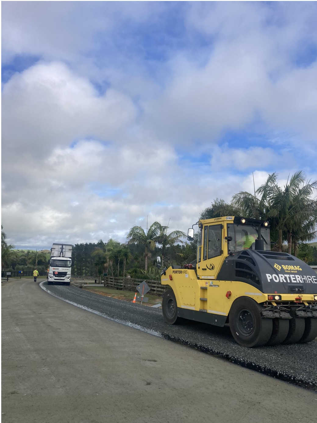
Taipa View Rd Rehabilitation – Sealing in Progress
