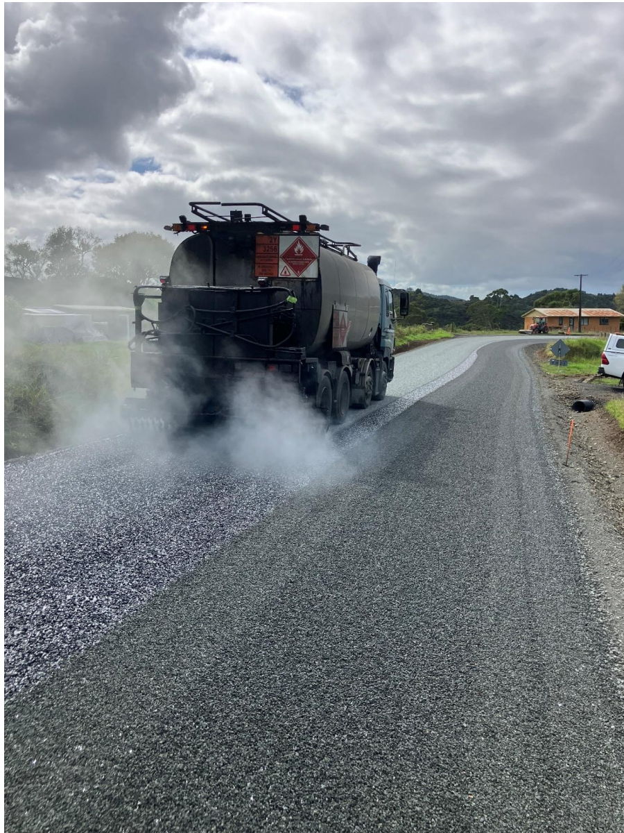
West Coast Rd Seal Extension – Sealing in Progress
