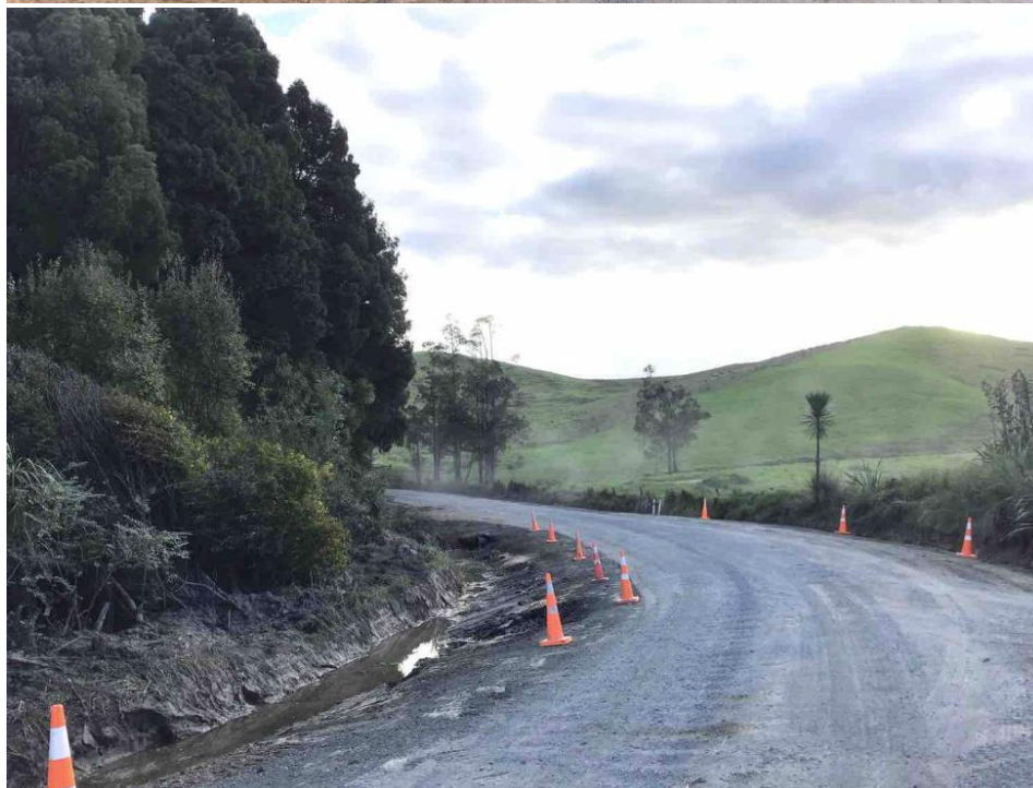
Peria Valley Rd – Water tabling and Clearing in Progress
