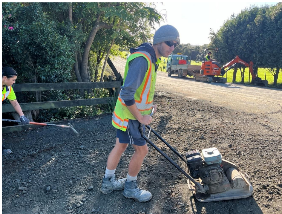
Driveway preparation on Larmer Rd Rehab
