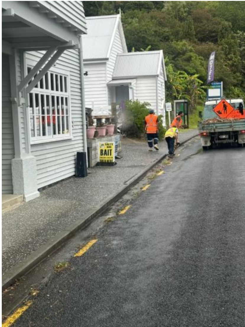
Kohukohu Rd - Kerb & Channel Clearing
