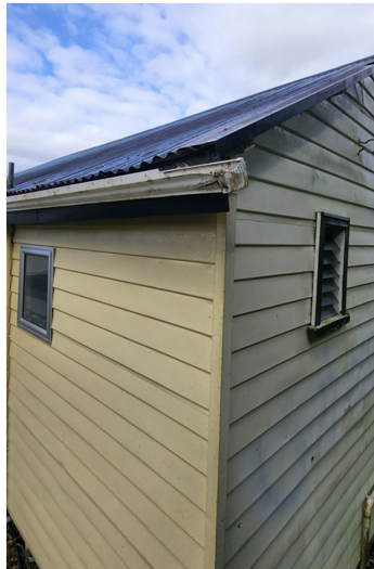
Damaged gutters
