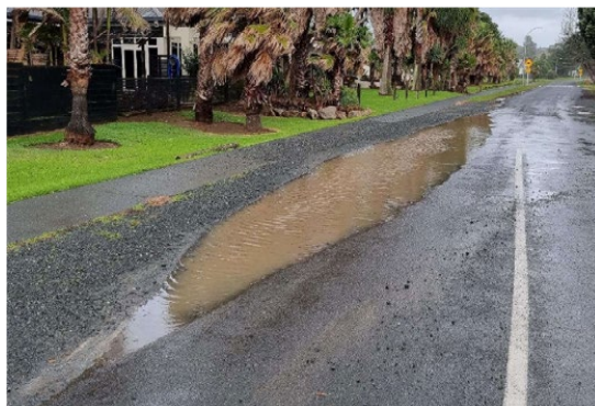
Figure 4a & 4b: Storm water & drainage issues.
