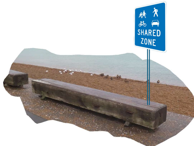
Signs mounted on timber baulks
