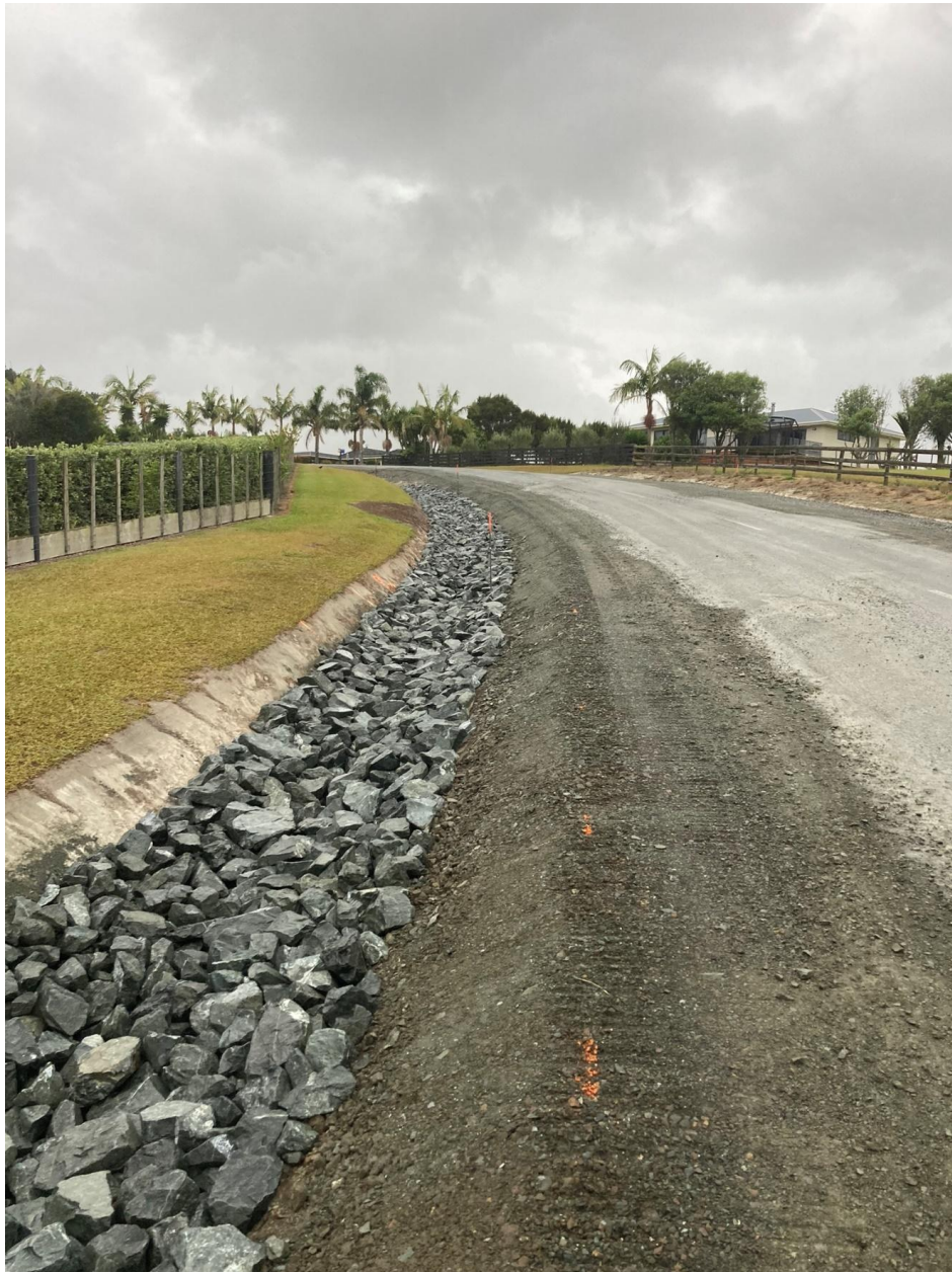
Taipa View Rd Rehabilitation – Rock rip rap scour protection and shoulder undercuts complete
