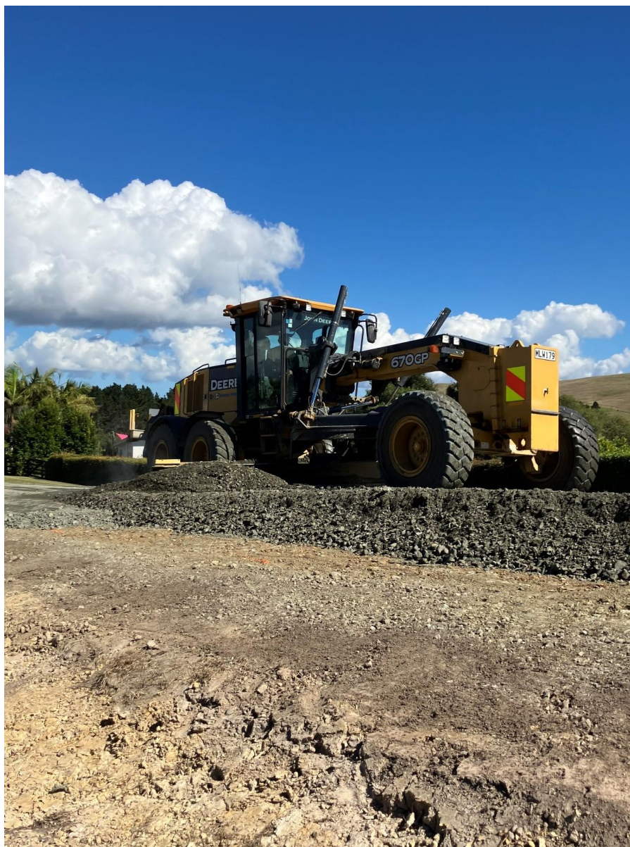
Taipa View Rd Rehabilitation – Shoulder undercuts in Progress
