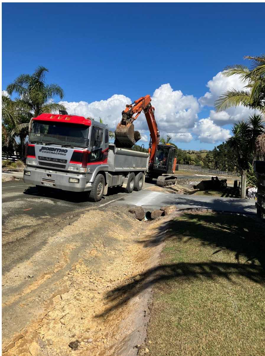
Taipa View Rd Rehabilitation – Concrete removal to allow for pavement overlay
