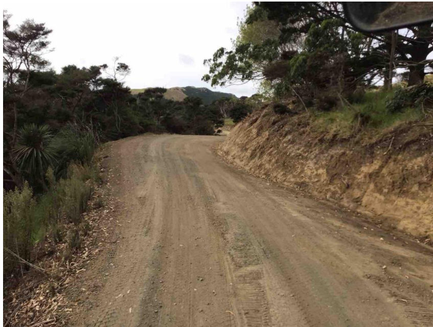
Owhata Rd – Water tabling and Clearing in Progress
