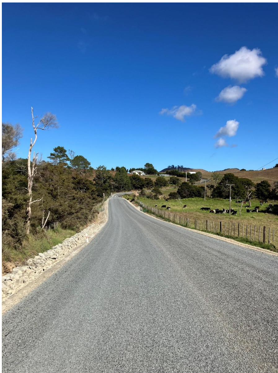
Taupo Bay Rd Rehabilitation – Sealing Complete
