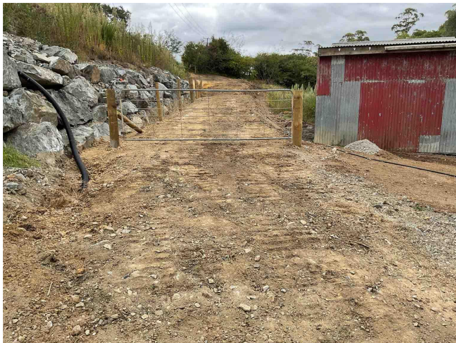
Fencing of the Ruaroa Rd Seal Extension Rock Spall Retaining Wall
