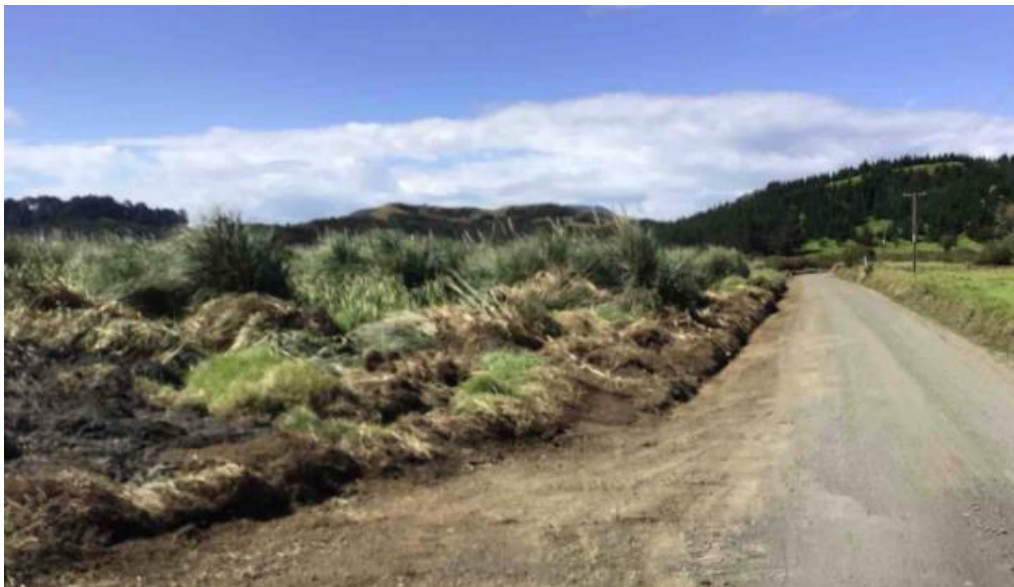
Owhata Road Watertabling in progress
