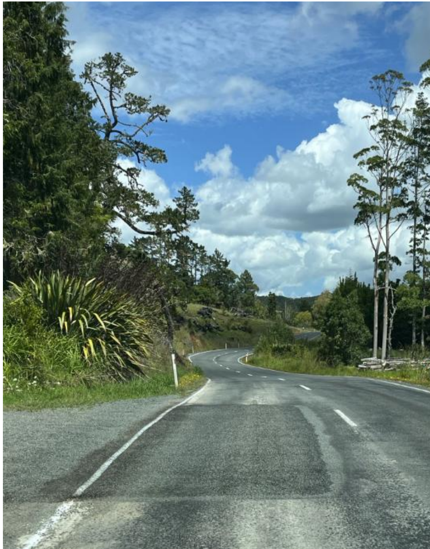
Oruru Rd Pavement Repair
