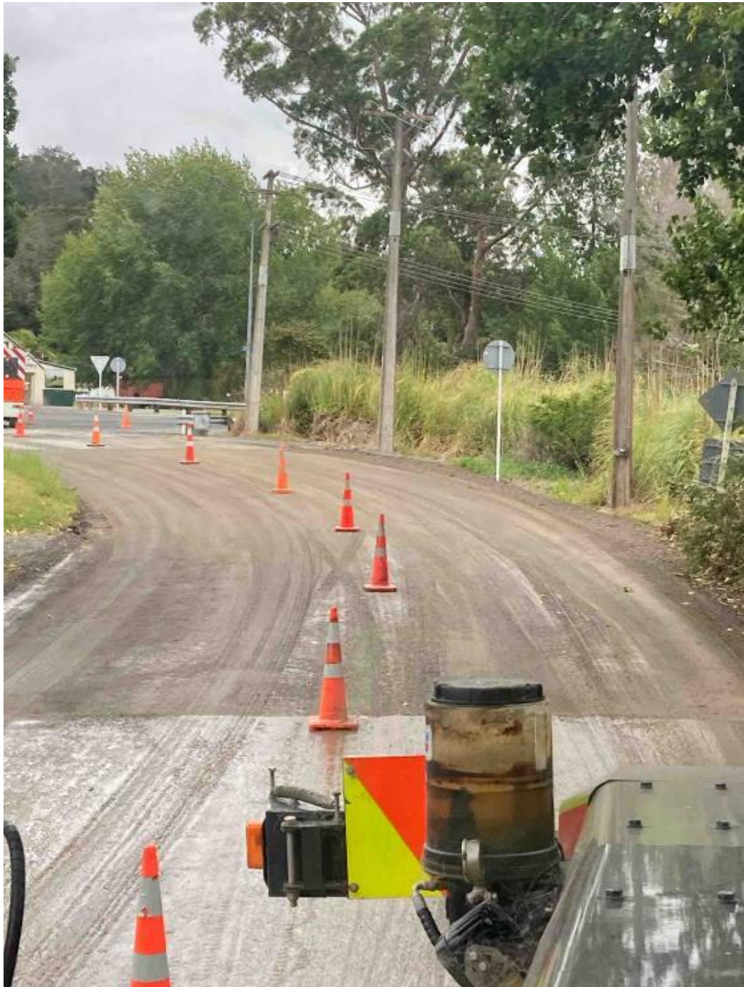
Duncan Road Pre Seal Repairs
