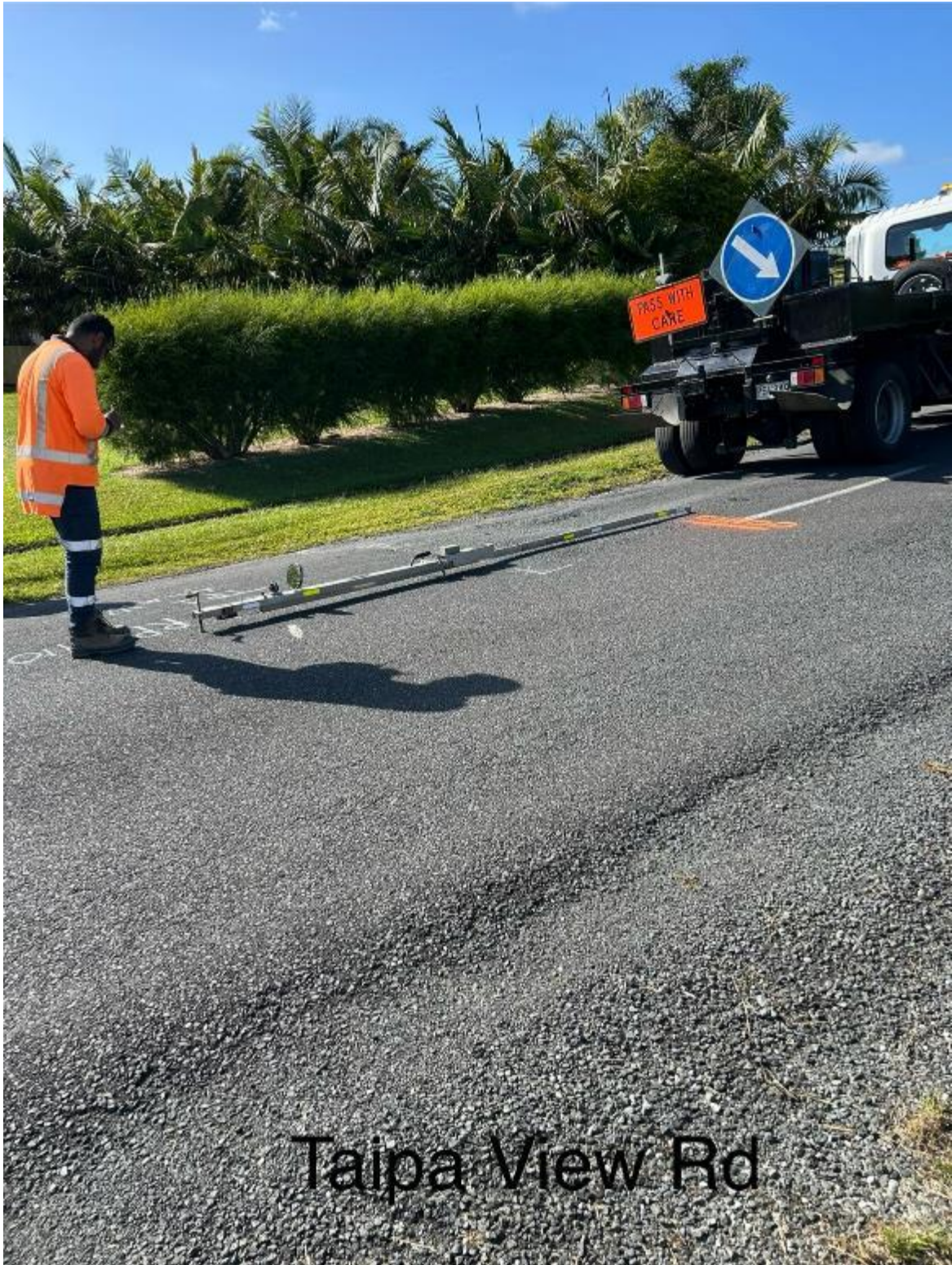
Beam testing Taipa View Rd
