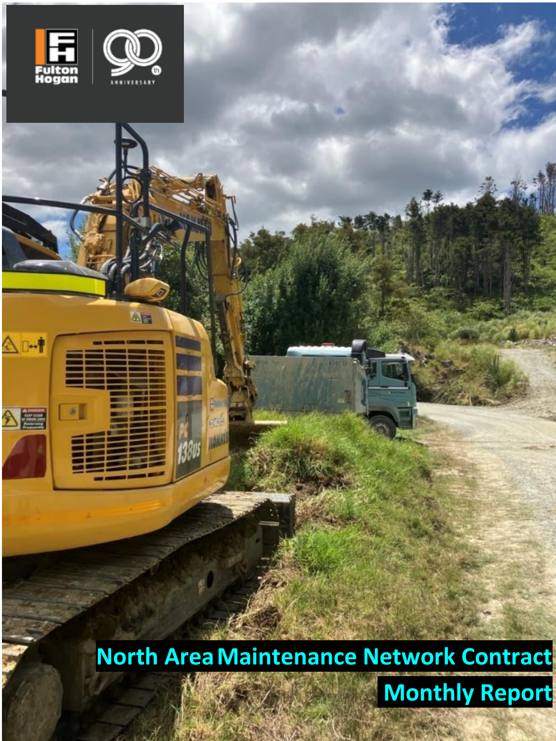
Contract 7/18/100 FNDC North Road Maintenance & Renewals
