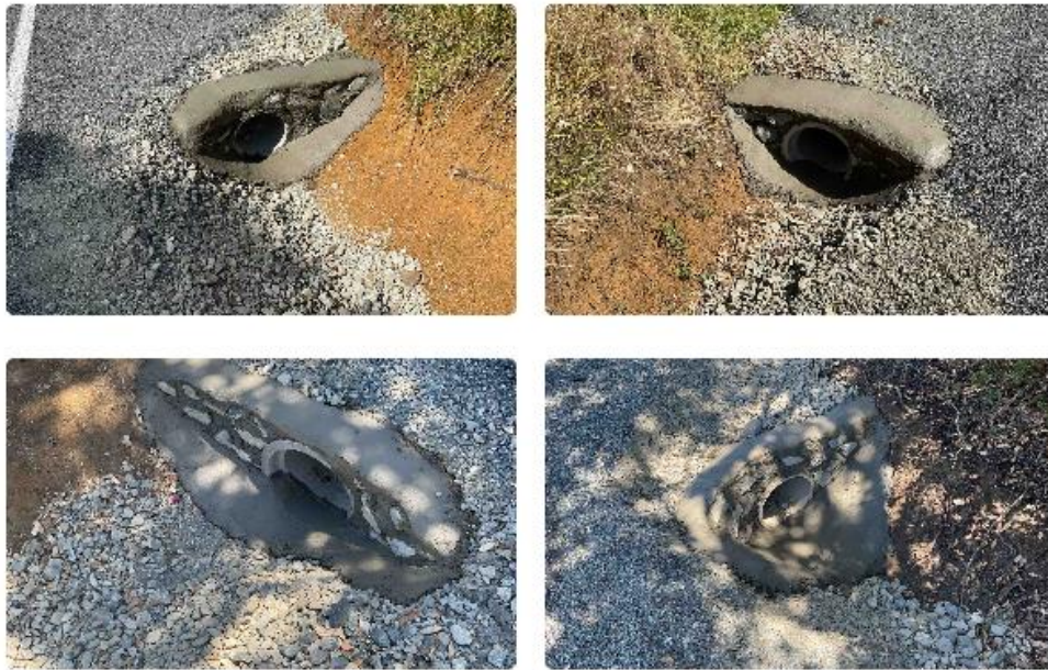
Headwalls Takahue Rd Rehab
