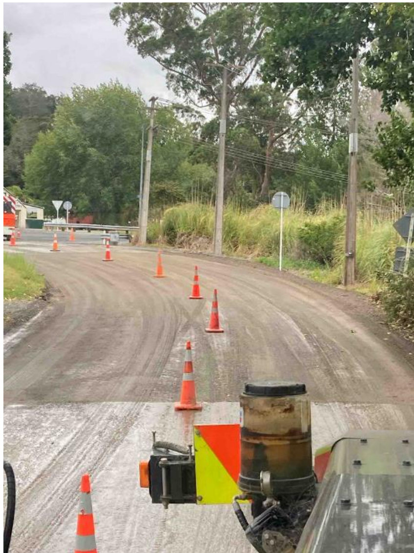
Duncan Road Pre Seal Repairs
