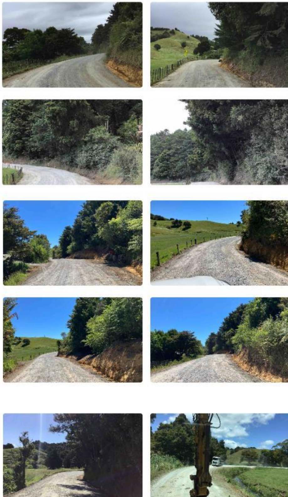
Water tabling in progress – Mangatoetoe Road
