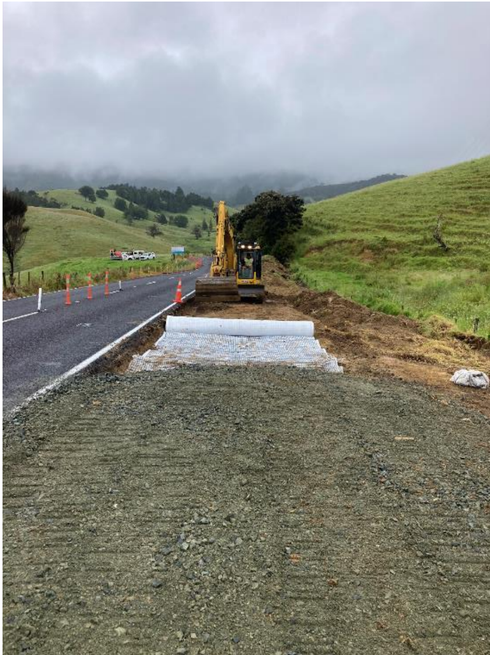
Wainui Rd Slip Repair Retreat in Progress
