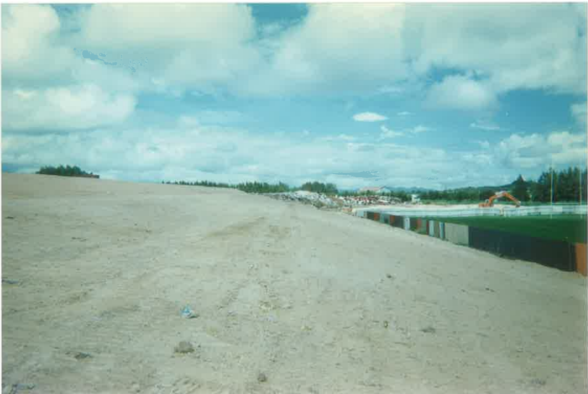
Viewing Terraces After Clay Capping
