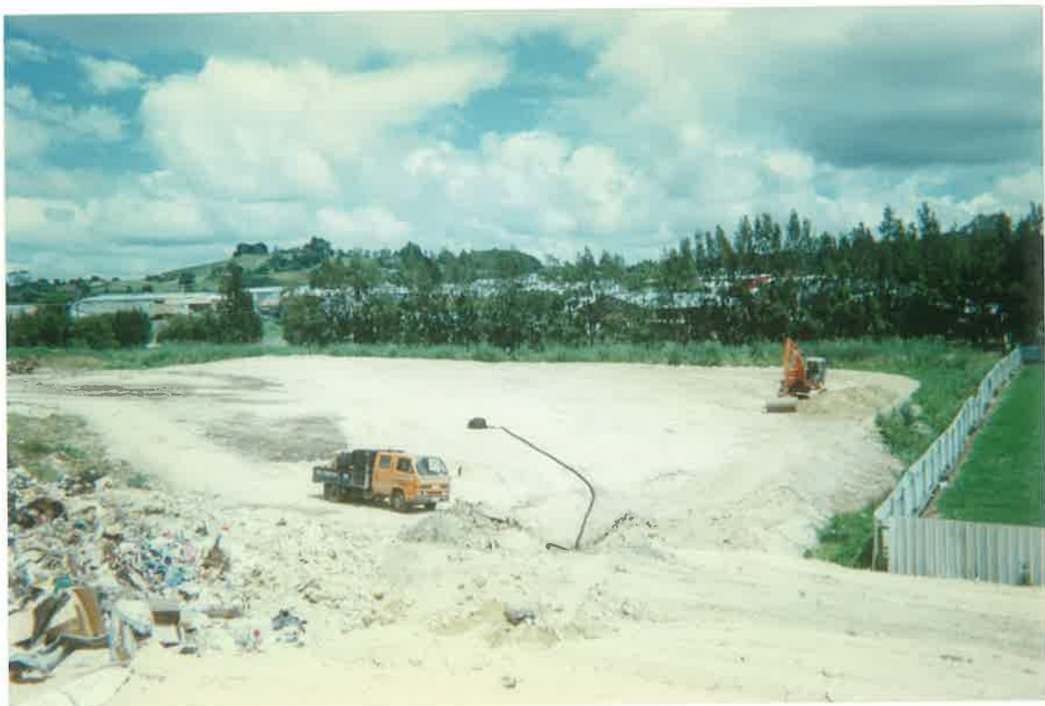
Preparation Of Liner For New Area
