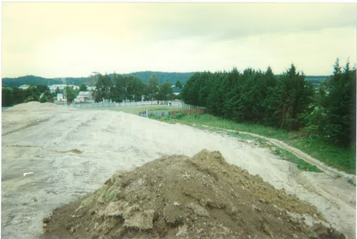
Batter Slope Clay Capping Eastern Boundary (Concrete Lined Swale Drain)
