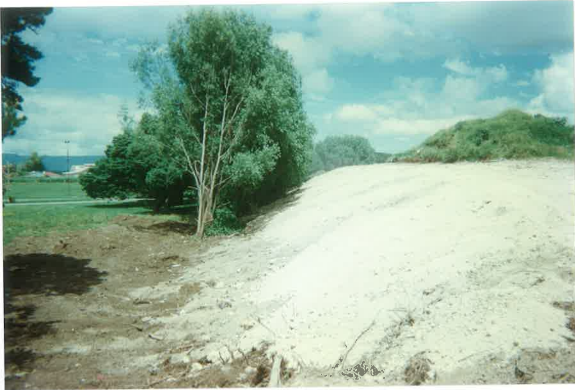
Willows Removed & Clay Capping In Progress On Southern Batter Slope (Note: Topsoil Stockpile On Landfill Crown)
