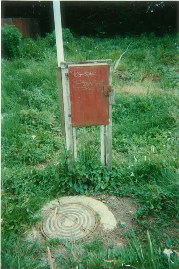
Leachate Pump Chamber With Telemetry Chamber
