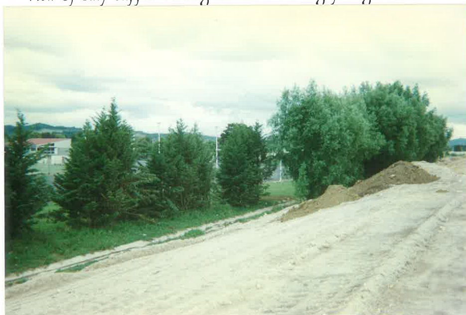
View Along Eastern Batter Slope. Willow Trees Are Being Progressively Removed As Clay Capping Proceeds
