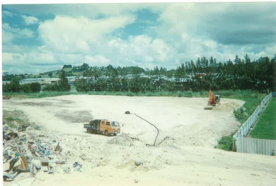
Preparation Of Liner For New Area
