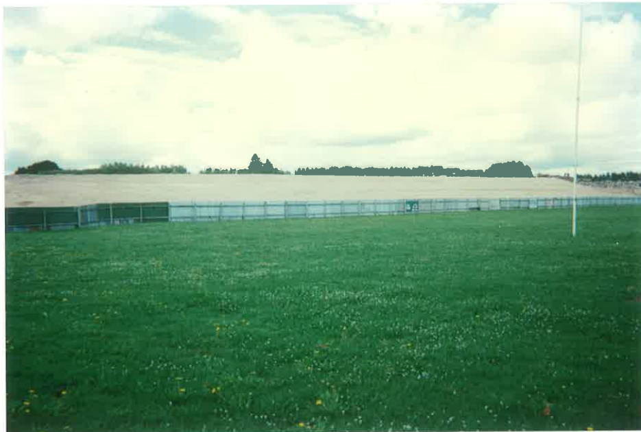
View Of Clay Capped Viewing Terrace From Rugby League Field
