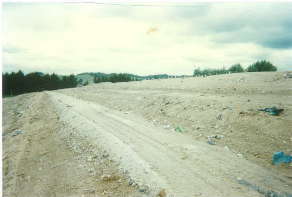
Viewing Terrace Prior To Clay Capping
