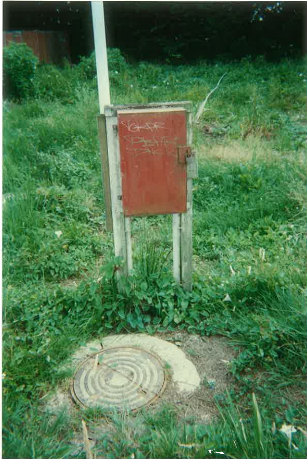
Leachate Pump Chamber With Telemetry Chamber
