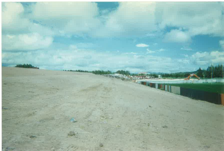
Viewing Terraces After Clay Capping
