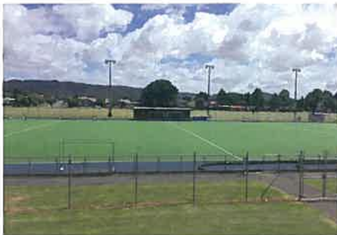
3. Hockey turf including lighting and fencing
