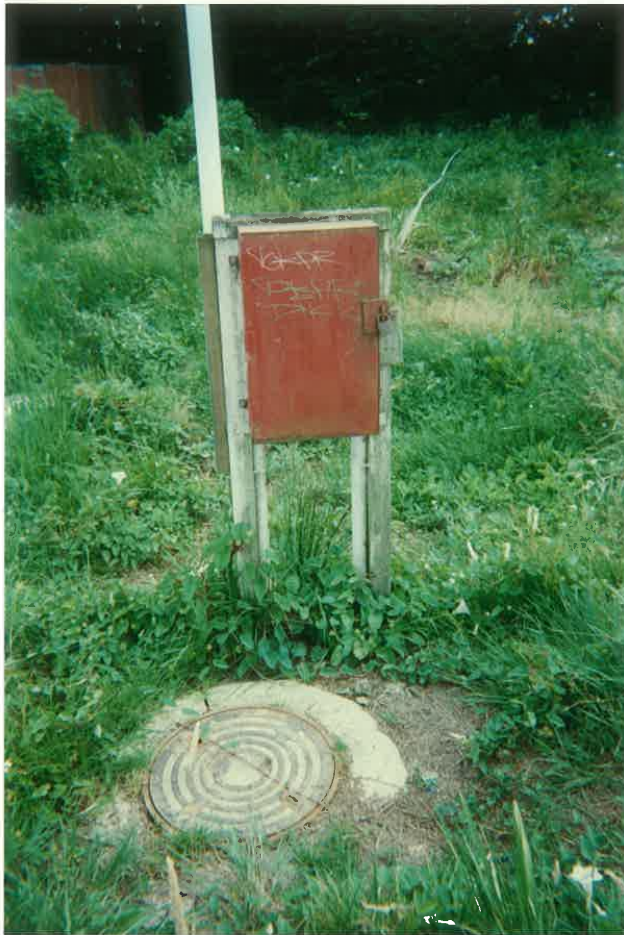
Leachate Pump Chamber With Telemetry Chamber
