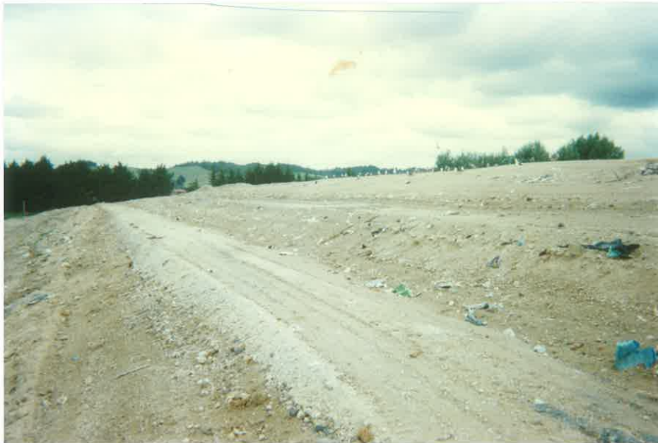
Viewing Terrace Prior To Clay Capping
