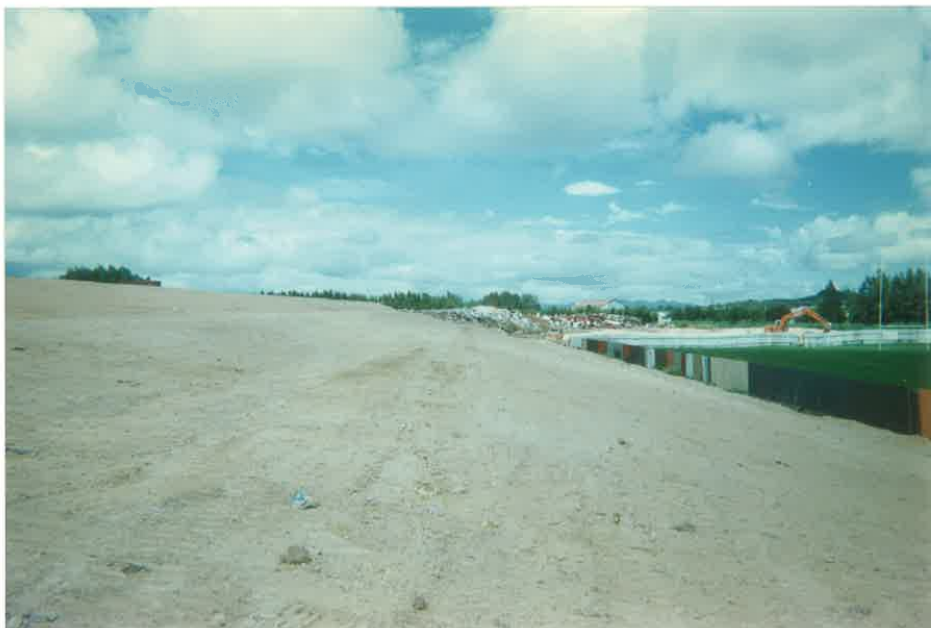
Viewing Terraces After Clay Capping
